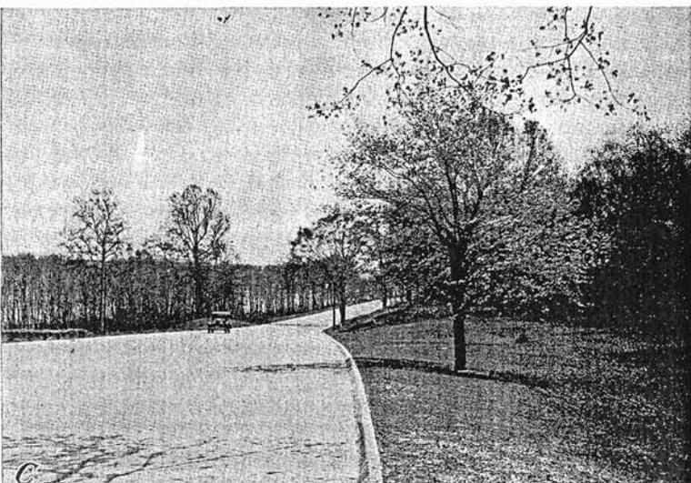
COMPLETED PROJECT. NOTE LOCATION TO FIT NATURAL CONTOURS, ROUNDED SLOPES, ABSENCE OF DITCHES, RUSTIC GUARD RAIL AND RESULT OF SELECTIVE CUTTING. GROUND IS SEEDED BUT SOD NOT YET ESTABLISHED.
