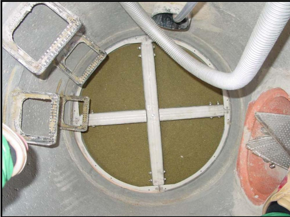
**Figure 27:** Filter unit equipped with clinoptilolite as a barrier material (Technical University of Munich).
