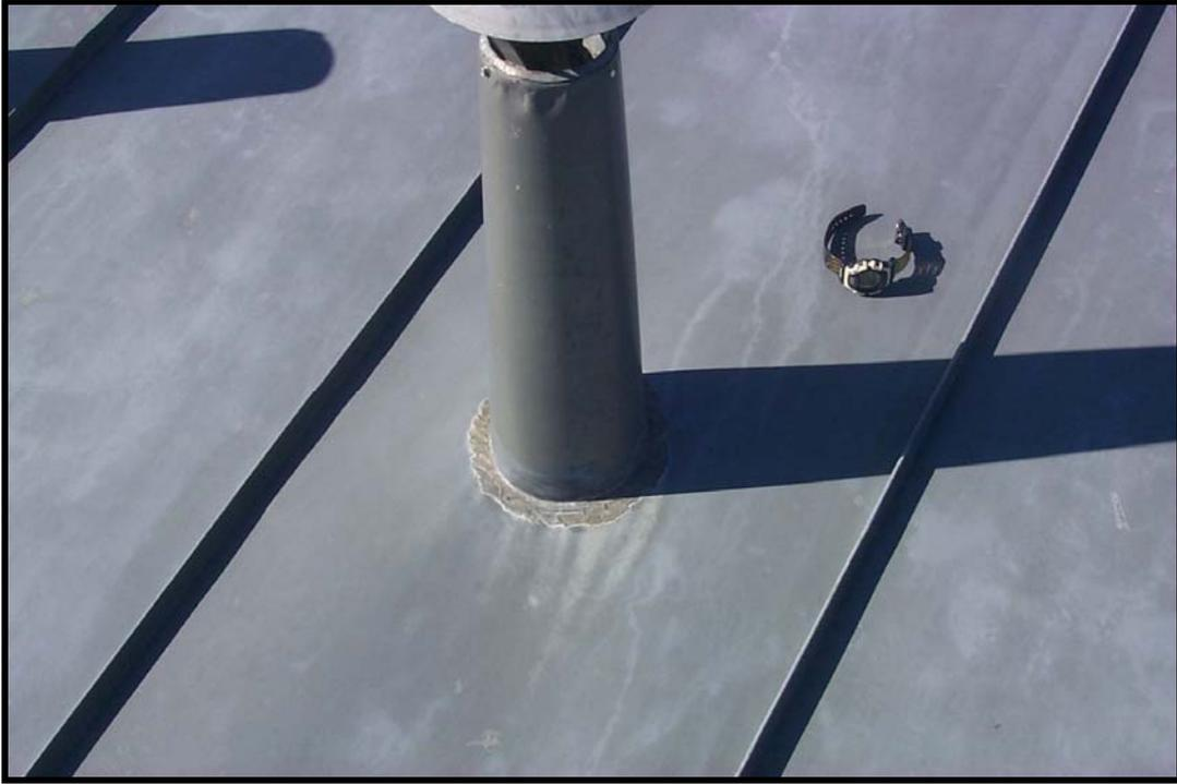
**Figure 67:** Photo from the antimony-free solder sealing material used to seal the chimneys on the roof.
