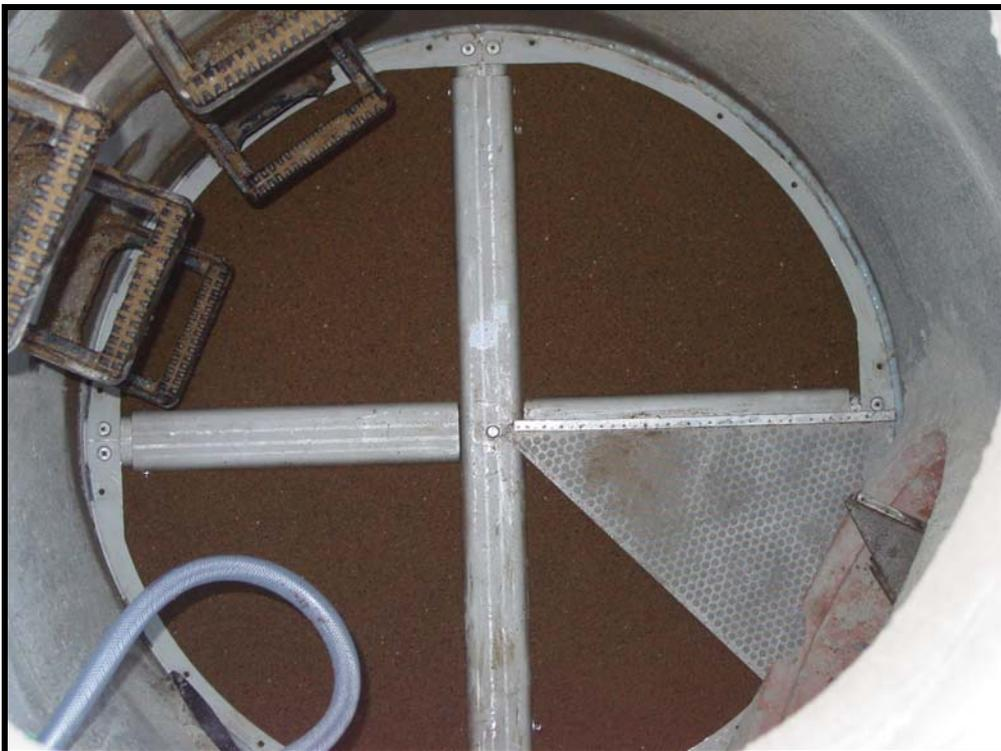
**Figure 26:** Filter unit equipped with a mix of chabazite-philipsite as a barrier material (Technical University of Munich).
