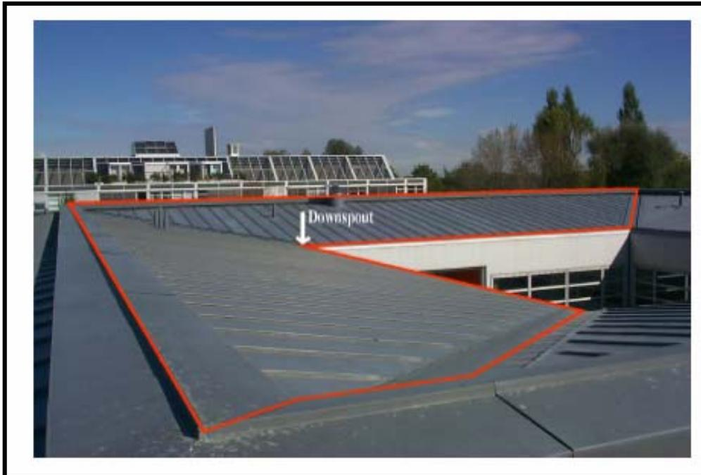
**Figure 17:** View of the zinc roof with its sampling surface.
