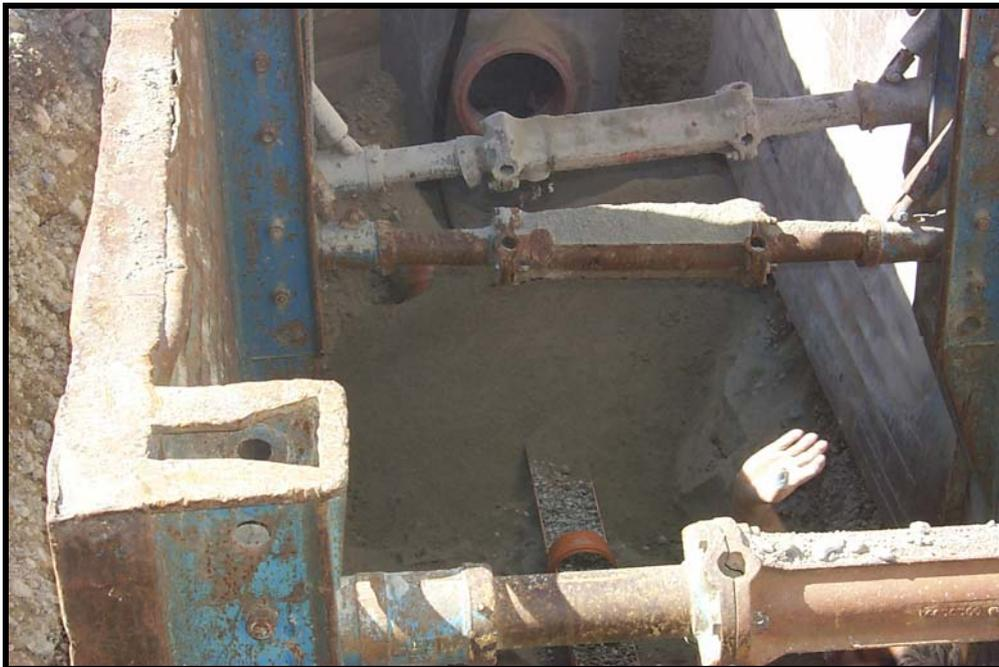
**Figure 28:** Installation of the sampling unit underneath the infiltration ditch.
