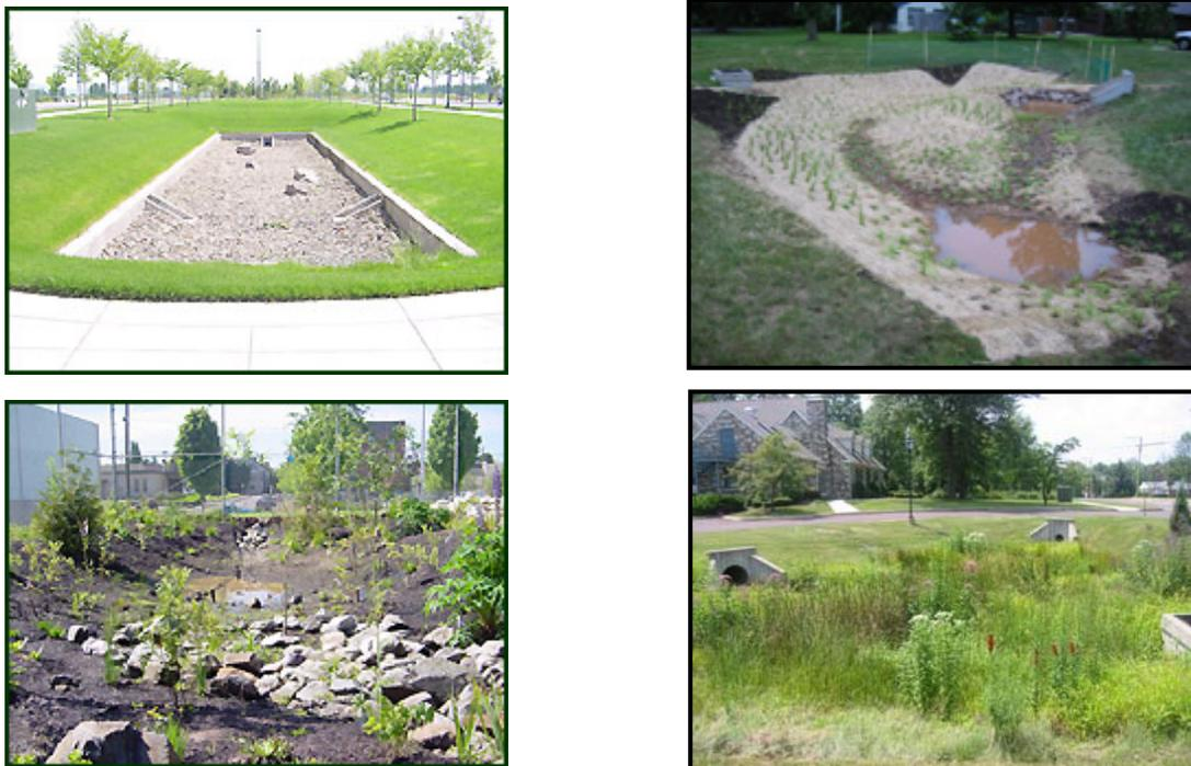
**Figure 12:** Pond, basin and constructed wetland for storm water treatment.
