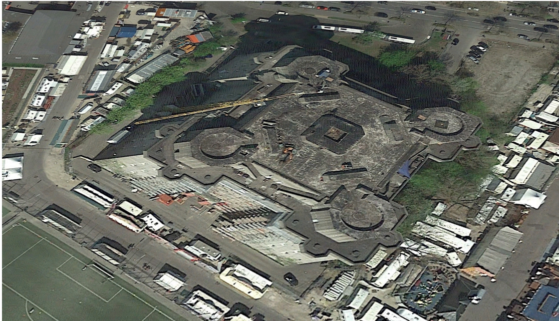
(a) Before construction work in 2019
