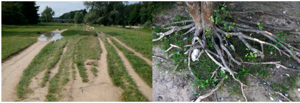
Fig. 6. Picture of the vegetation damages observed. Left: trampling trails. Right: root breakage. (For interpretation of the references to colour in this figure legend, the reader is referred to the web version of this article).
