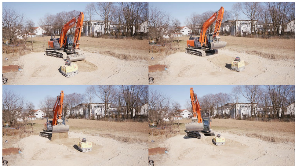
Fig. 18 Testing of the collaborative compaction process on a German construction site
