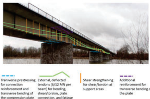
Figure 3: Overview of the strengthening concept for BK60
