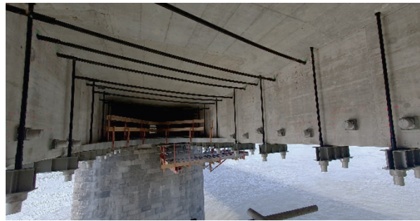
Figure 11: View into the box girder area field 8
