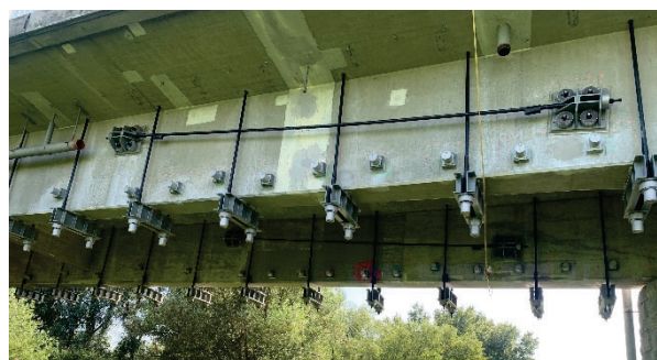
Figure 12: Longitudinal prestressing at the coupling joint 1
