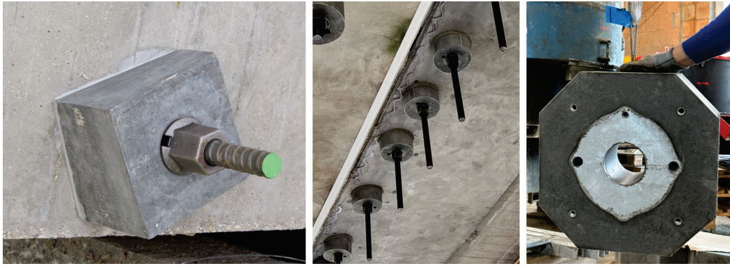
Figure 4: HA for bars SAS 1050 47WR with double inclination ( left ); HA-Round for bar Macalloy 1030 32 mm ( center ); HA for FB 98 mm ( right )
