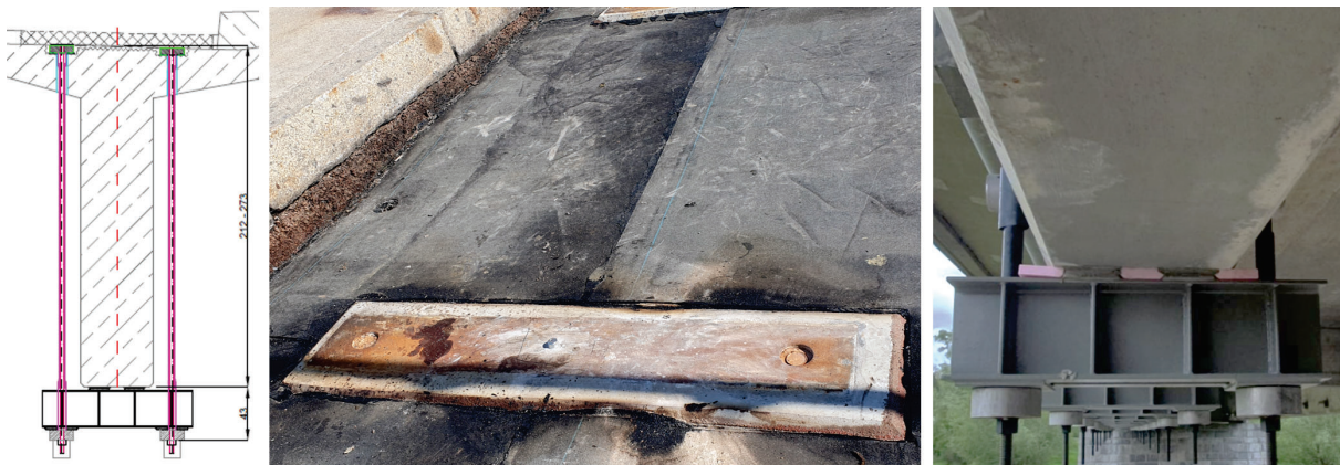
Figure 12: Cross-Section of the pt system ( left ); threaded ended plate with 1,5 m length ( middle ); steel crossbeam with HA plates ( right )
