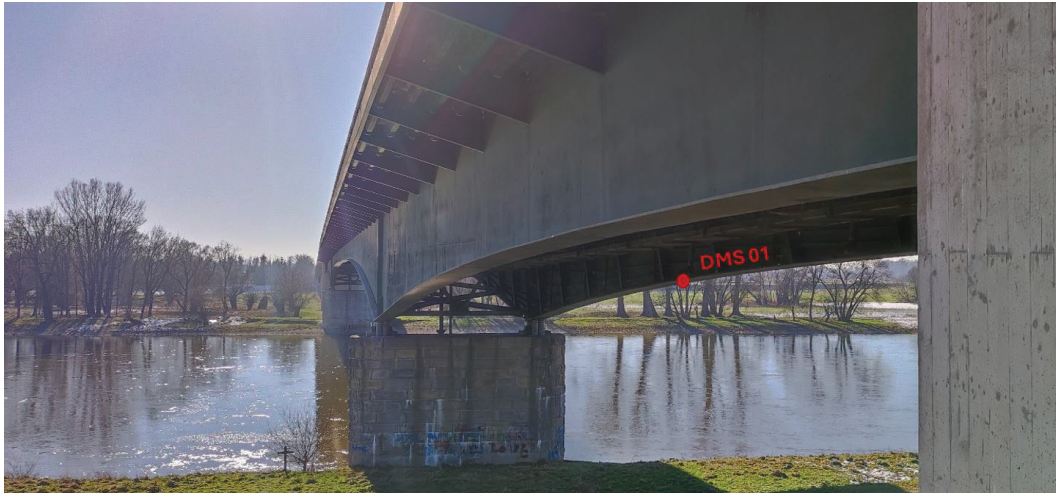
Figure 2: Danube bridge Winzer (seen from the abutment Winzer to pier P6)
