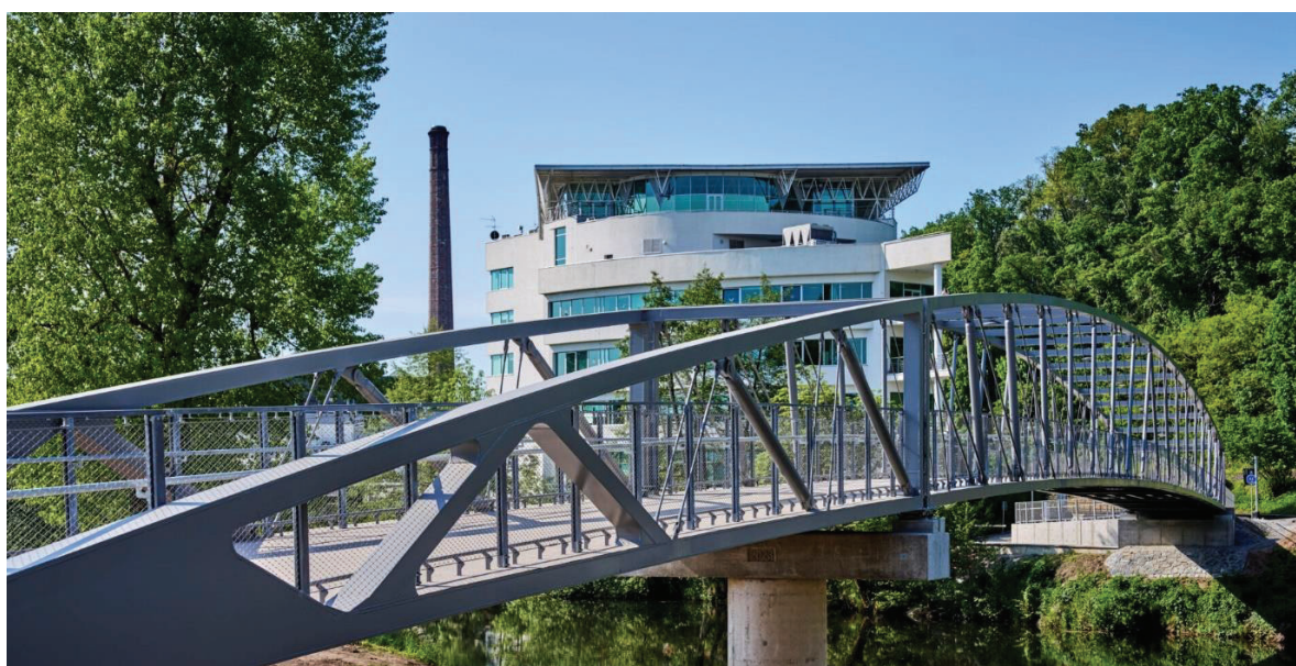
Figure 5: Footbridge in Mladá Boleslav, CZ (Source: Škoda auto, 2023)
