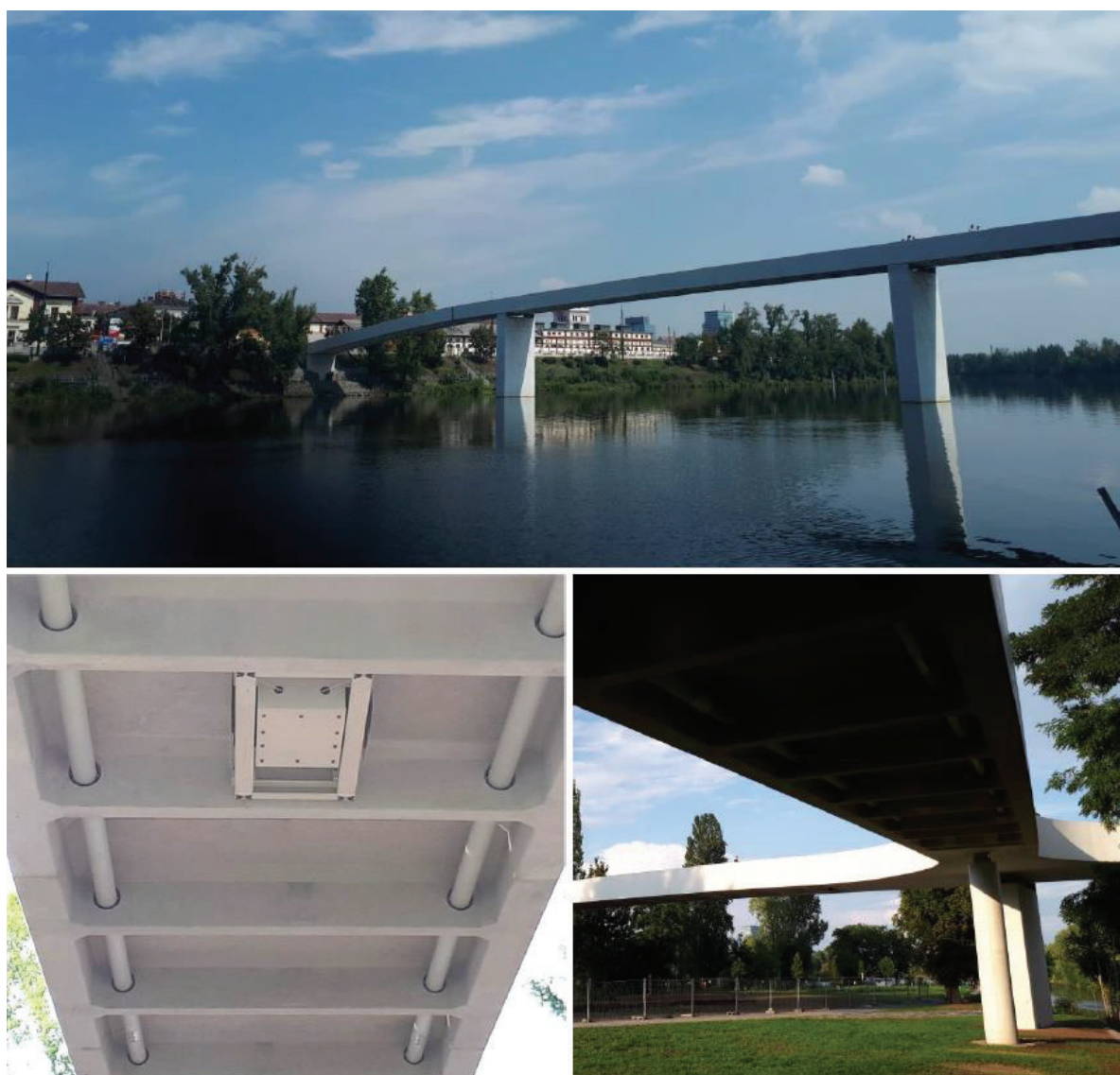
Figure 6: Štvanice Footbridge in Prague, TMD from KGF hydraulika, Island Štvanice, CZ
