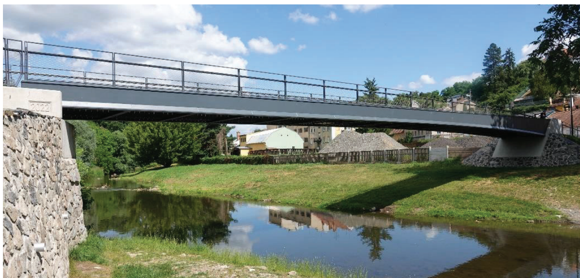
Figure 3: Footbridge in Bílovice nad Svitavou, CZ
