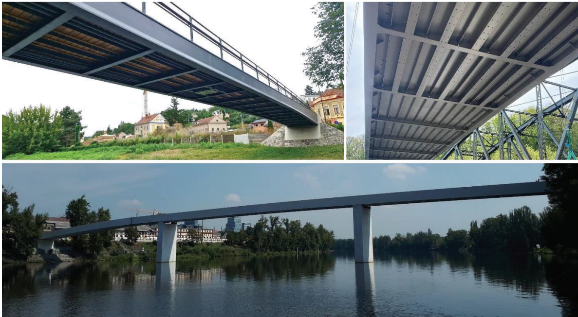
Figure 2: Challenges: flat bridge deck profile (footbridge in Bílovice nad Svitavou, CZ) – bridge deck with densely embedded girders (footbridge in Mladá Boleslav, CZ) – integration regarding form & function (Štvanice footbridge in Prague)
