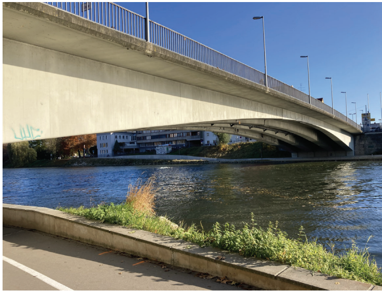
Figure 2: Bridge by Finsterwalder, source: author
