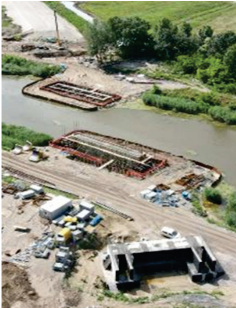
Figure 4: Construction site during the substructure work
