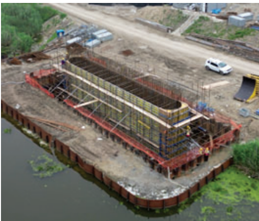
Figure 6: Execution of the middle column S3 in the cofferdam
