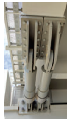
Figure 15: Shock transmitter unit
