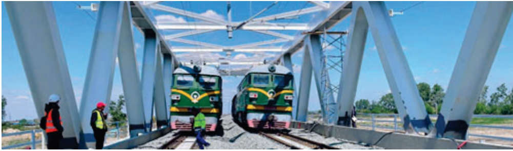
Figure 16: Photography at the time of bridge testing
