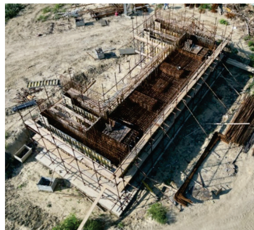
Figure 7: Execution of the abutment S4
