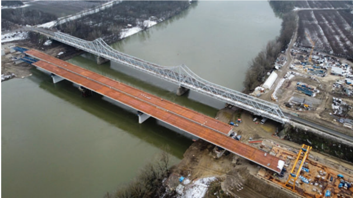
Figure 3: Assembly of the main bridge structure
