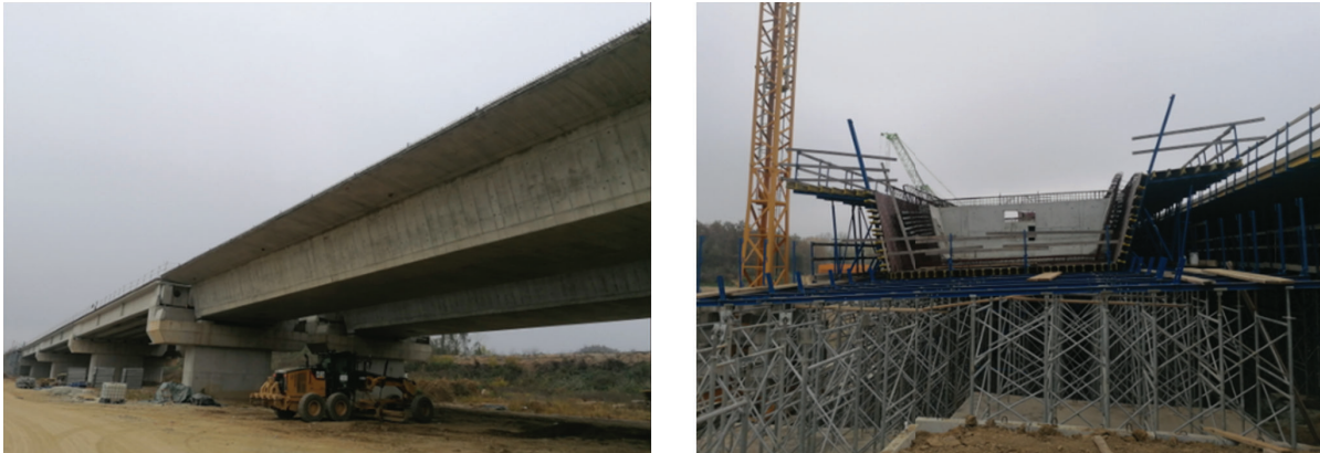
Figure 5: Box girder structures
