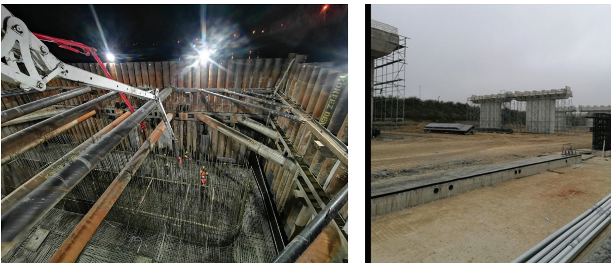
Figure 8: Piers of the main and access structure
