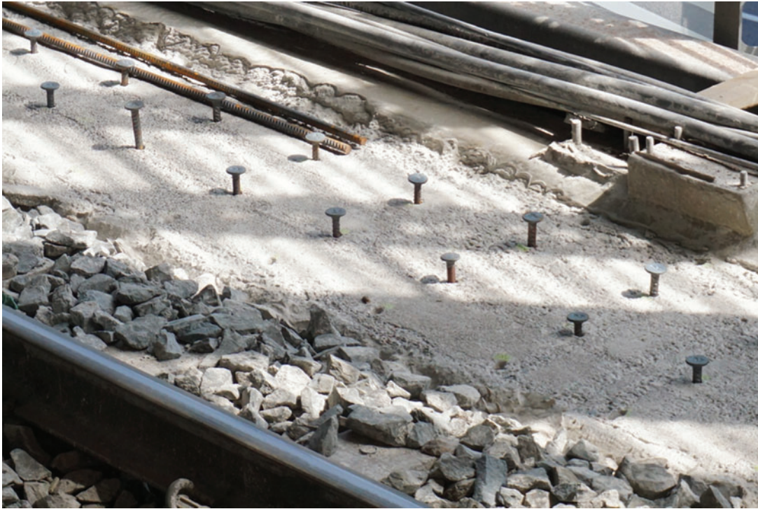
Figure 5: PSB® Headed bars use in bridge overlay, Helsinki 2022
