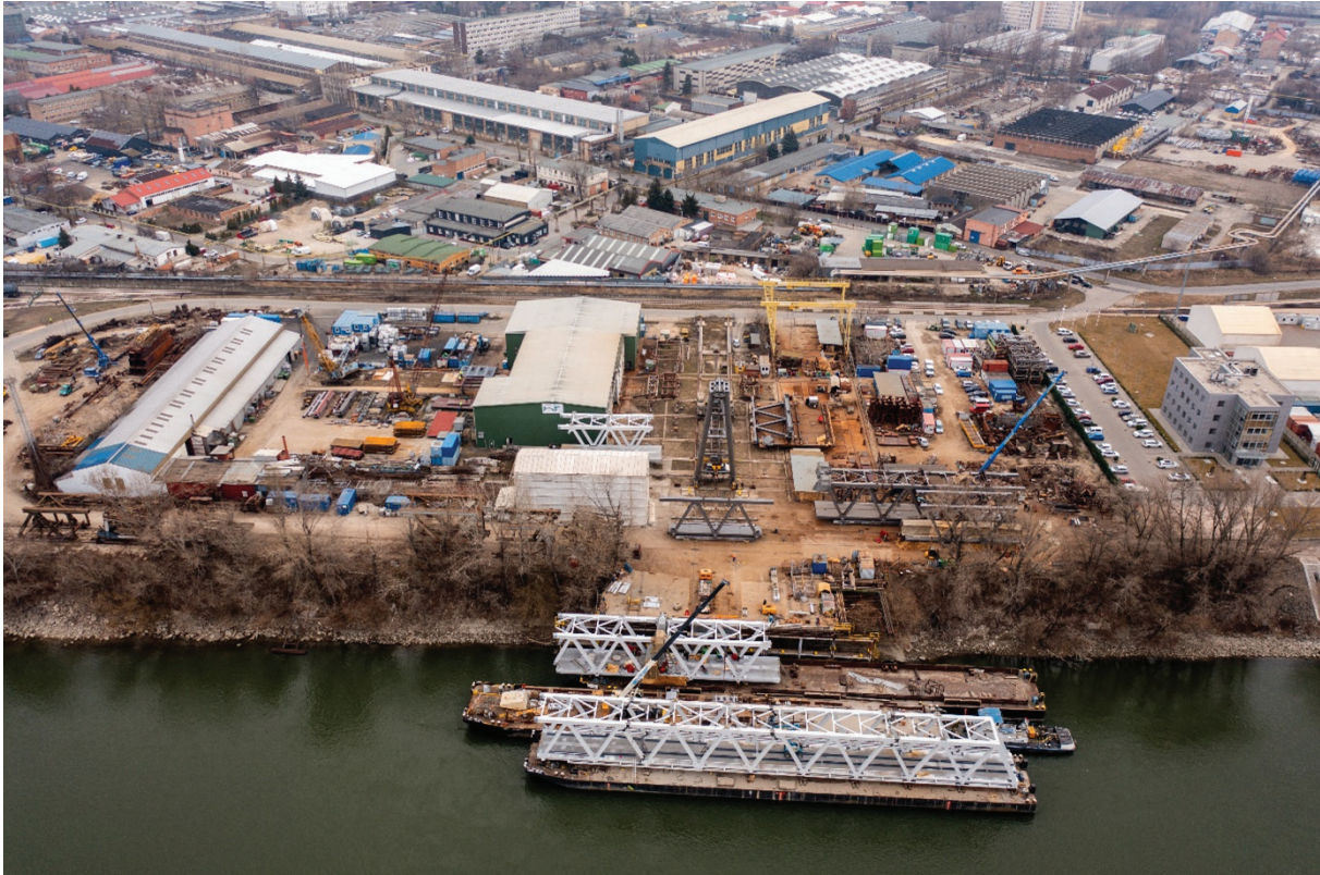
Figure 3: Pre-assembly a demolition area
