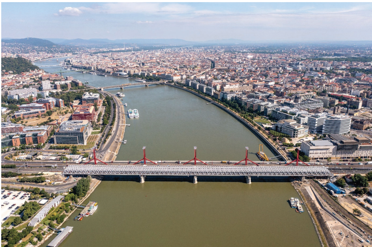
Figure 7: Despite being a railway bridge, it blends well into the cityscape
