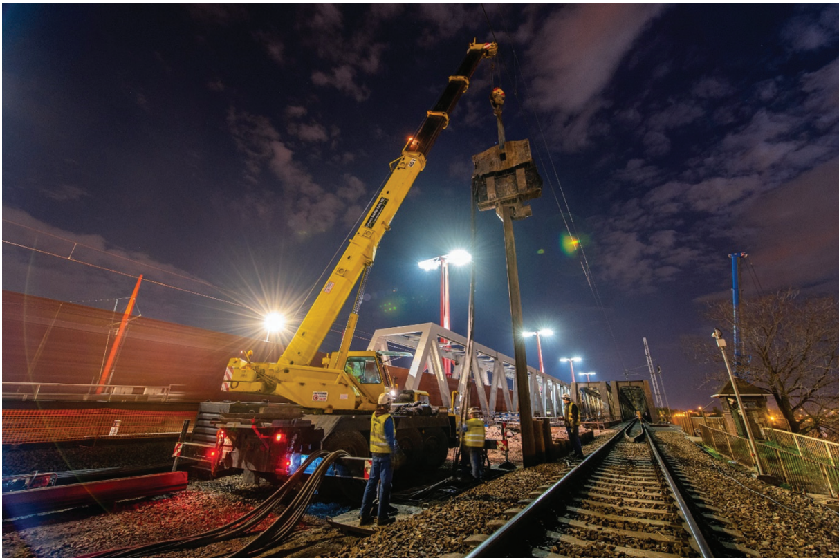
Figure 2: preparation of the abutment construction
