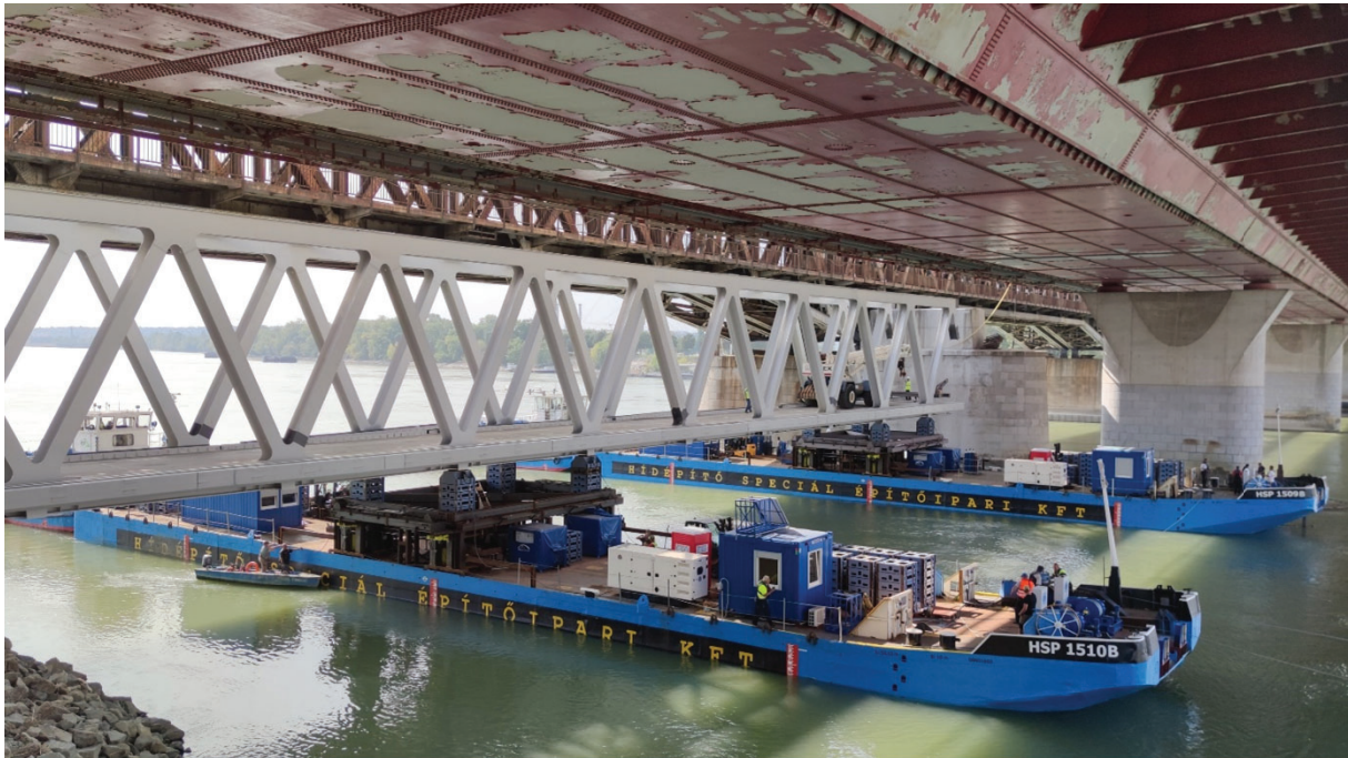
Figure 4: Heavy lifting equipment designed and built for this project
