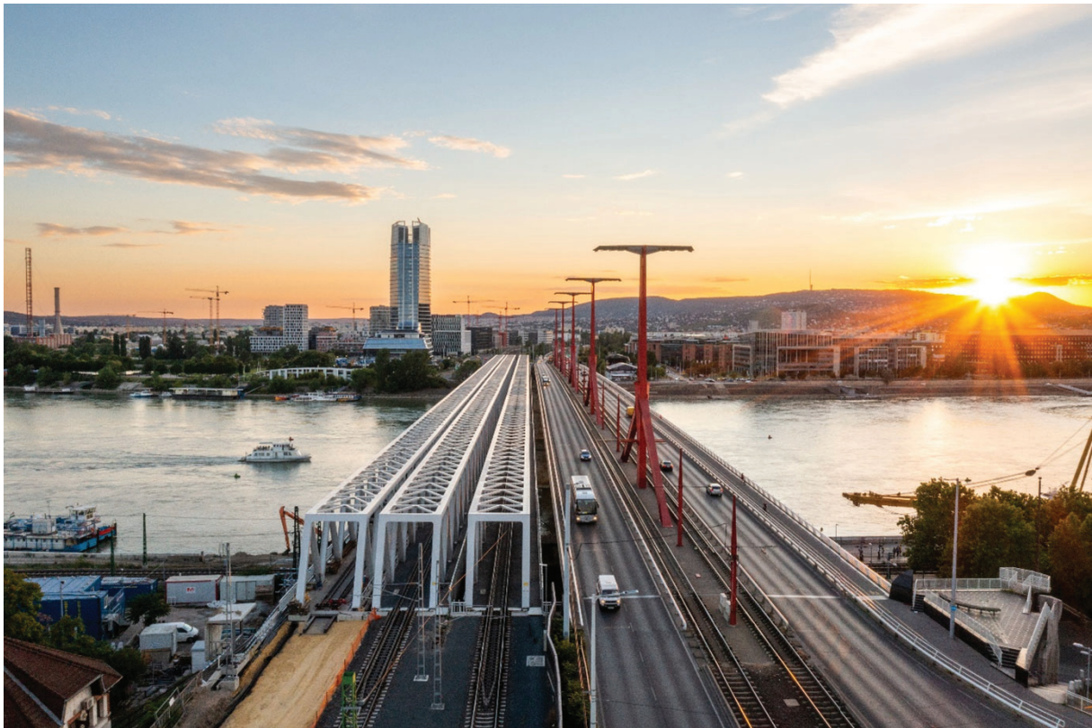
Figure 6: The three new bridges
