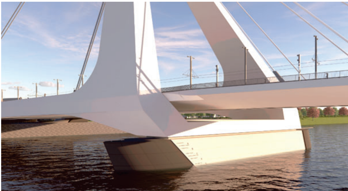
Figure 13: Rendered image of the final variant river pier and pylon structure – © UNStudio
