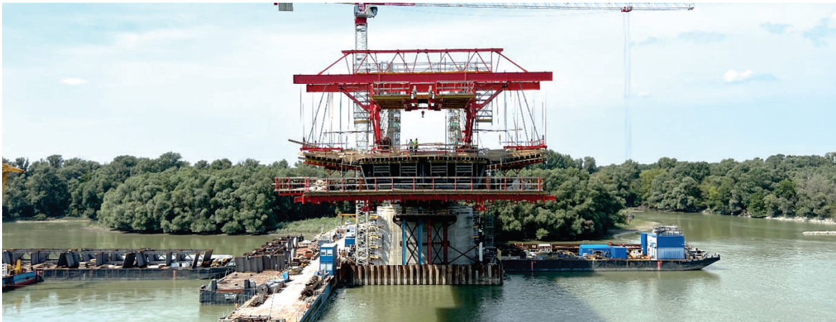
Figure 4: Balanced cantilever and form traveller – © CÉH
