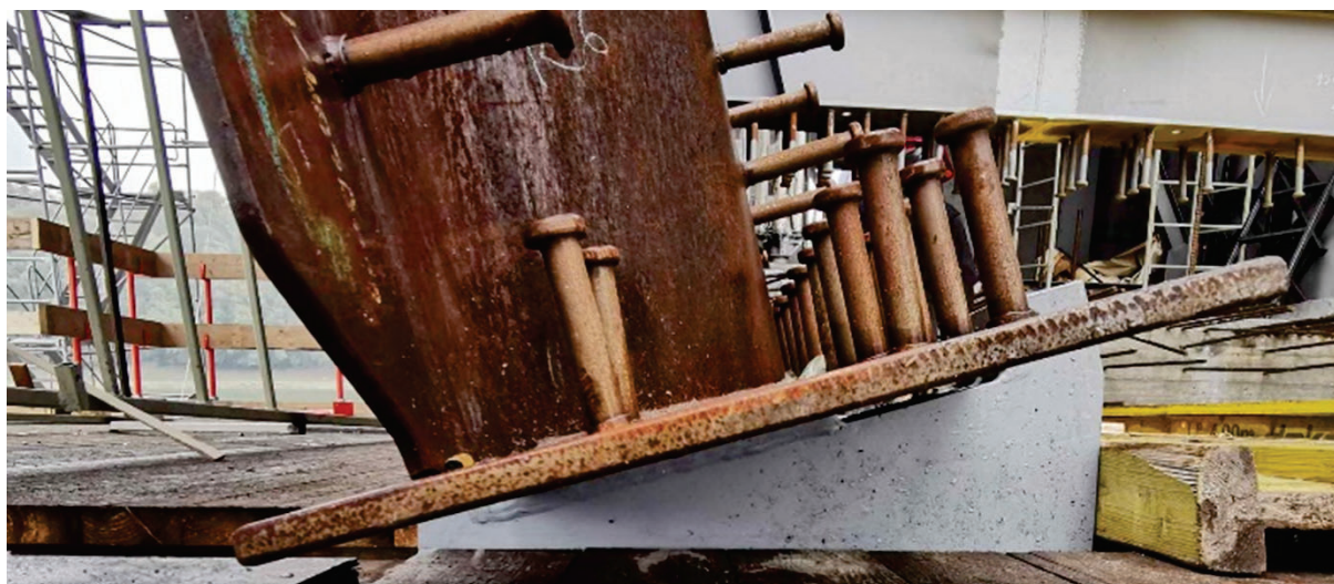
Figure 8: Transversal adjustment of the outer webs – © CÉH
