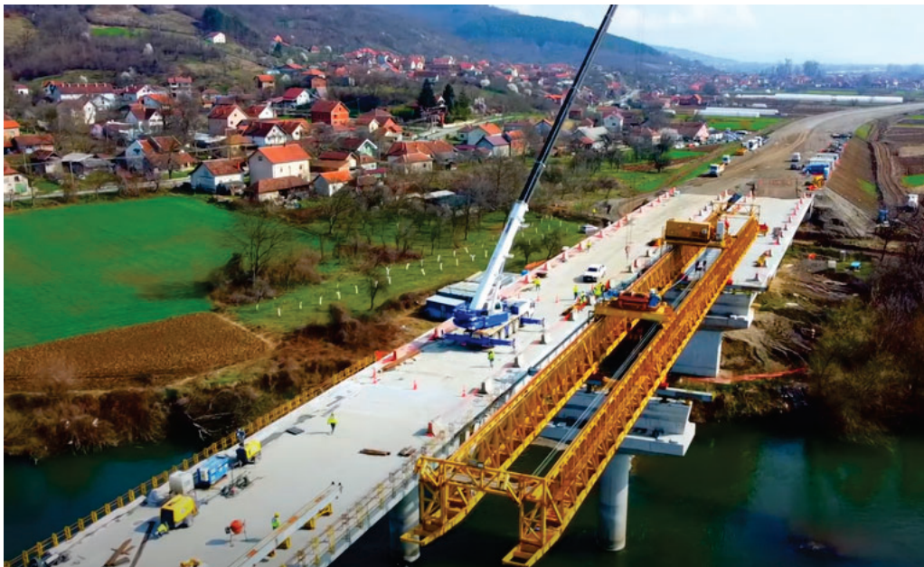
Figure 5: Erection of U-shaped precast beams with the launcher [4]
