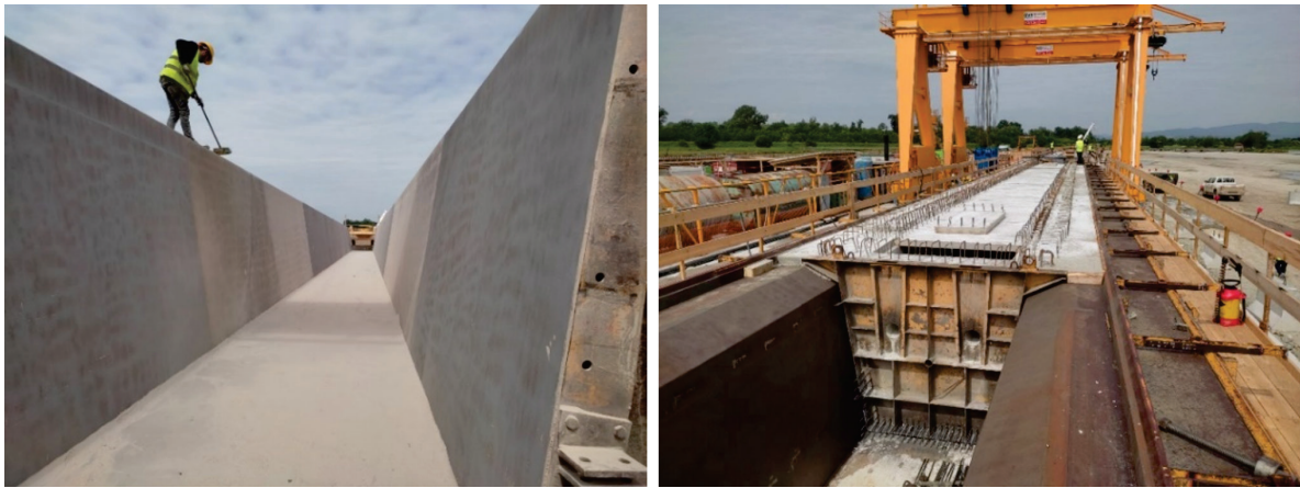
Figure 4: Casting of the U-shape precast beam
