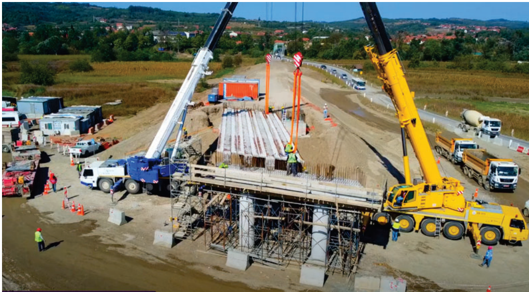
Figure 7: Erection of T-shape precast beam [4]
