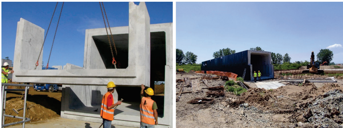
Figure 8: RC box precast culvert
