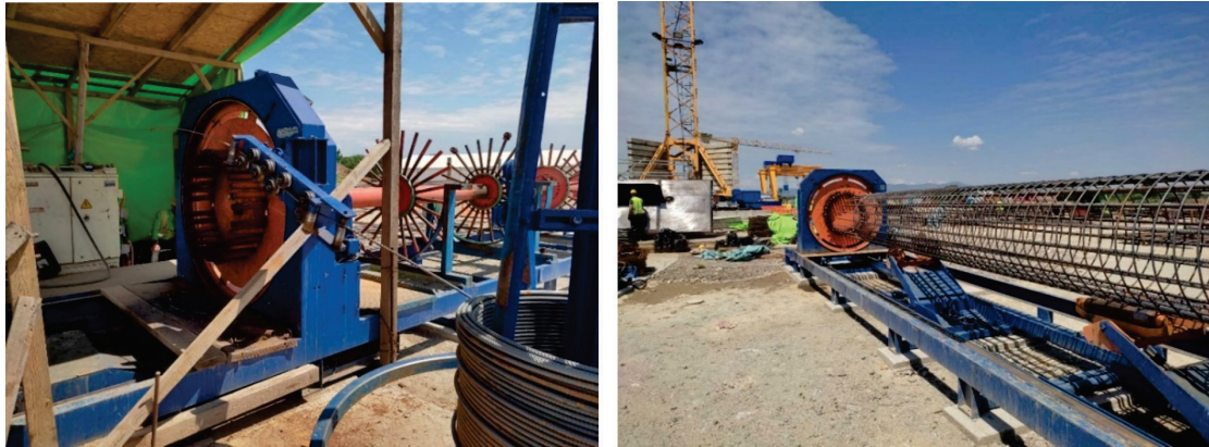
Figure 1: Equipment for pile rebar cage assembly
