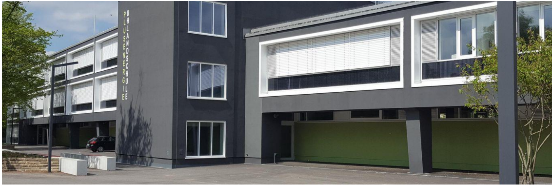
Figure 3-3: Uhland school building. View from the South East on the façade after the finished refurbishments. (Uhlandschule Zuffenhausen-Rot, n.d.)
