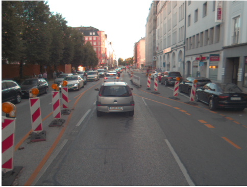
(a) Camera image from the Wiesn dataset. There are temporary lanes due to a construction site.
