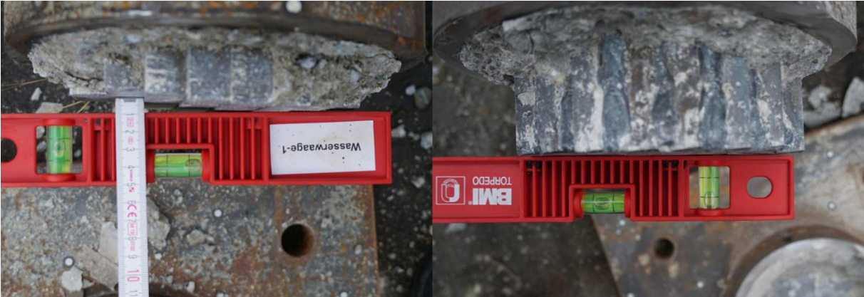
Figure 3-12 Relative displacement of the core profile (left KR-6, bolted; right KR-8, partially welded) [63].
