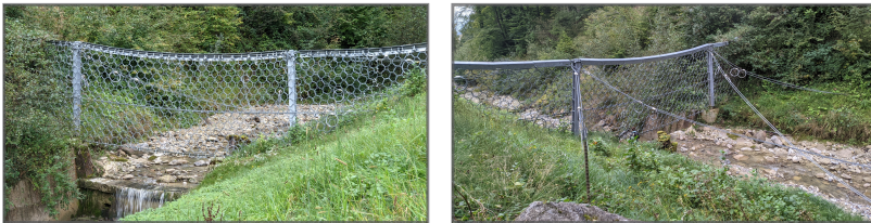
Figure 1.2: Flexible protective structure installed in Altstätten, Switzerland.
