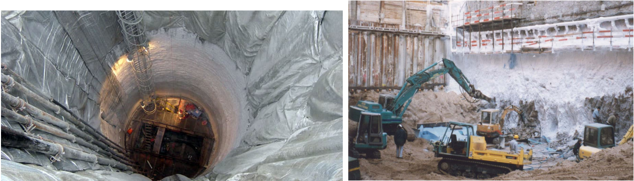
(a) Frozen soil body (white) supporting a shaft construction. Figure adapted from Tunnel Business Magazine (2024). (b) Frozen soil body (white) as a pit wall. Figure adapted from Orth (2014).
