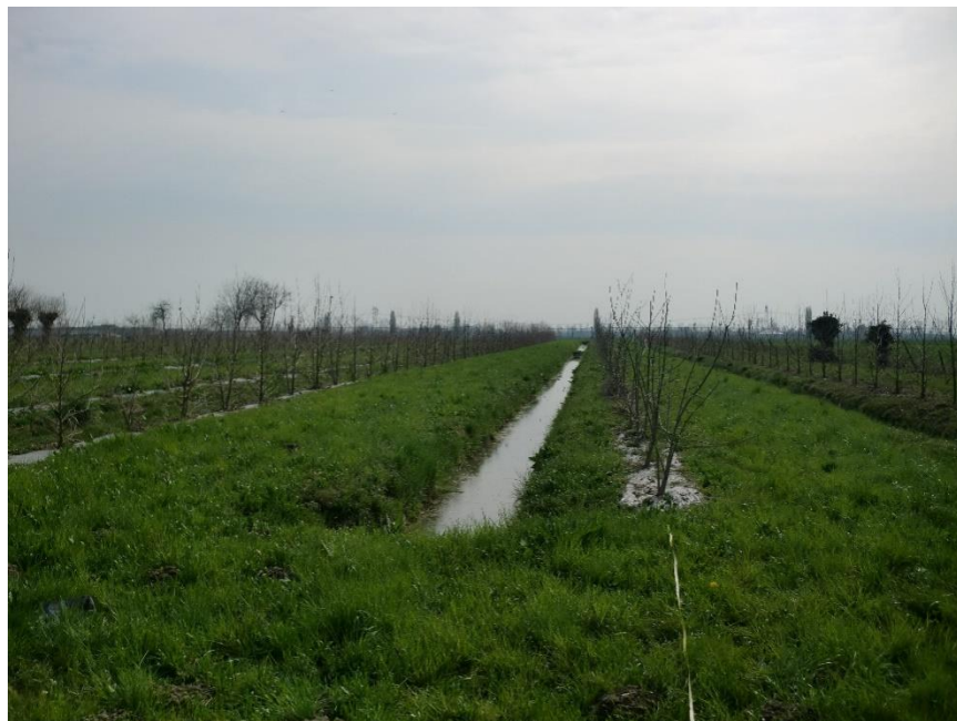
Figure 13 Infiltration trenches at Schiavon FIA.
