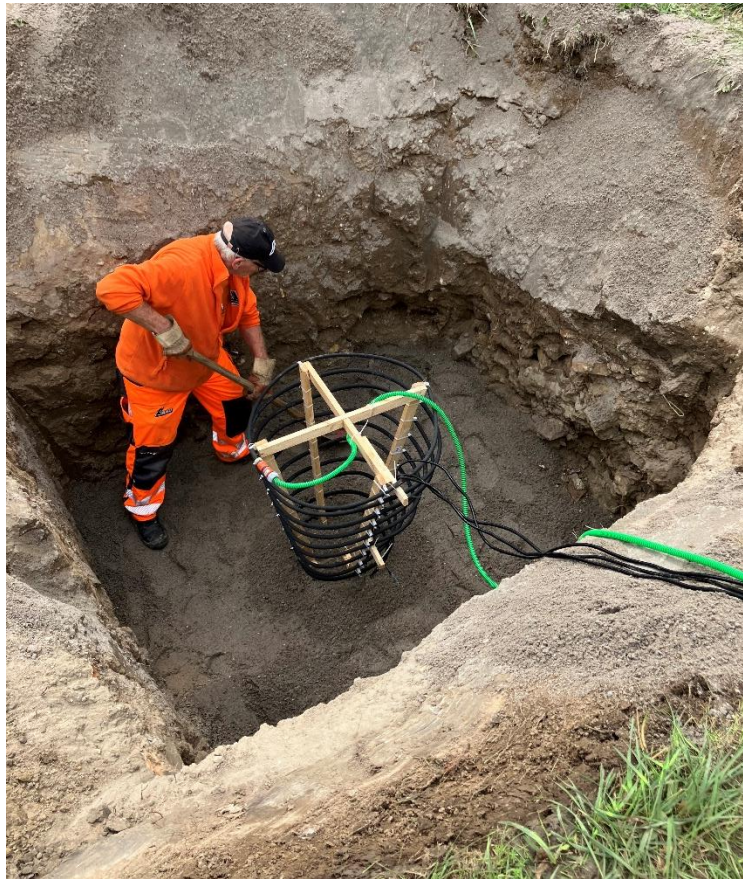
Figure 43 Installation of Prototype 2 at 2 m bgl.
