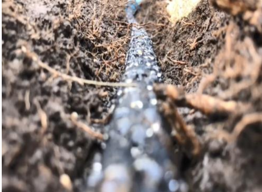
Figure 22 SIS used for aquifer recharge (Source: Ecotube).
