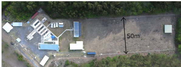
Fig. 1 Aerial photograph of the AGGO observatory. The area on the right side is reserved for the the new telescope.
