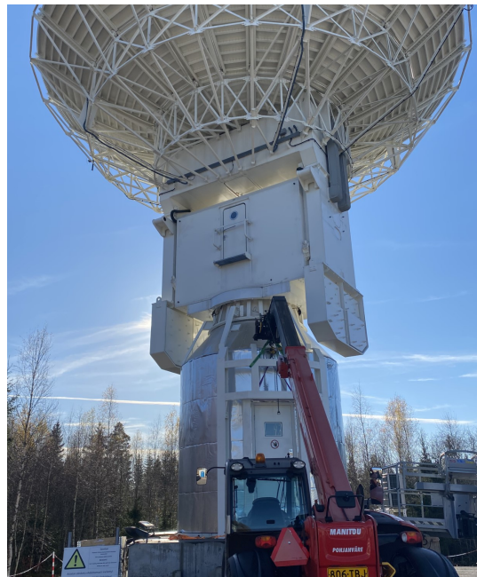
Fig. 2 Work on the telescope pedestal insulation (October 2022).
