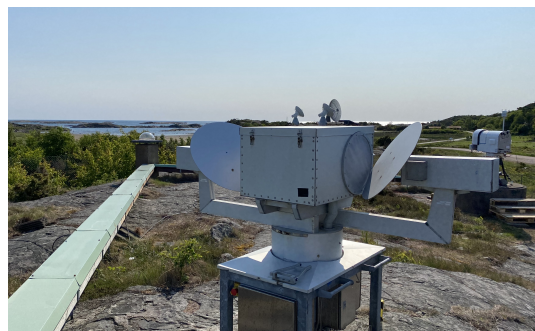
Fig. 1 The GNSS station ONSA (left, at the end of the cable tray) and the Water Vapour Radiometer (WVR) Konrad (in the foreground). The twin telescopes, and the 25 m radio telescope, are seen in the background. A new WVR (to the right), manufactured by RPG, was installed in May 2023, but has not been used in this study.
