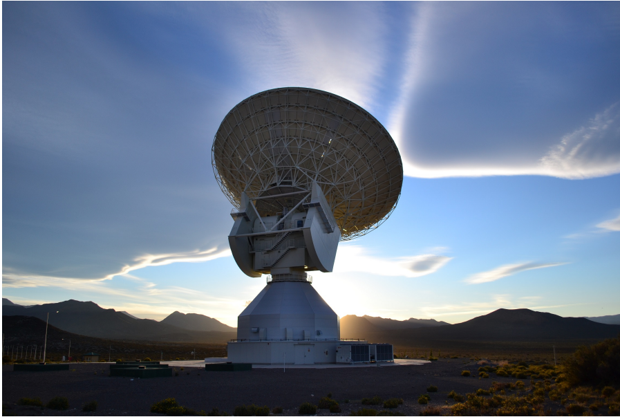
Figure 2.15: Malargüe Station Deep Space Communications Antenna. (© ESA/D. Pazos - CC BY-SA IGO 3.0)
