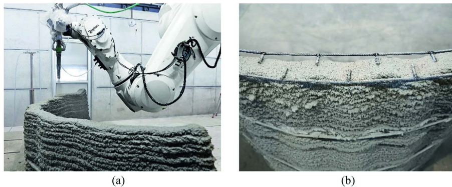
Figure 2.2: Shotcrete for wall building
