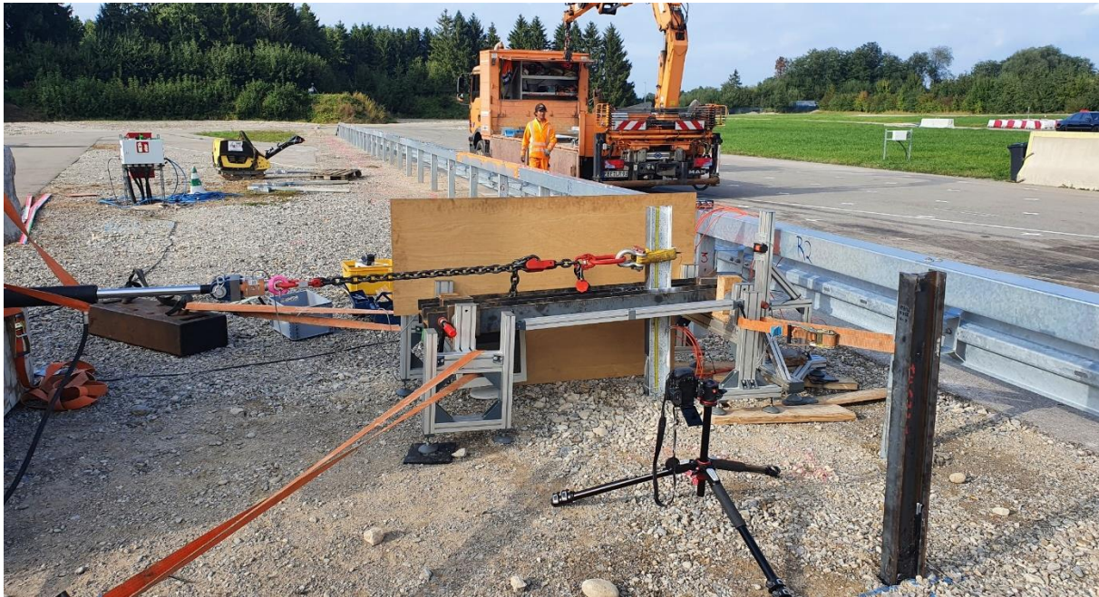
Fig. 3-17: Static loading test setup in-situ (IPE120 in GU055 crash test field)
