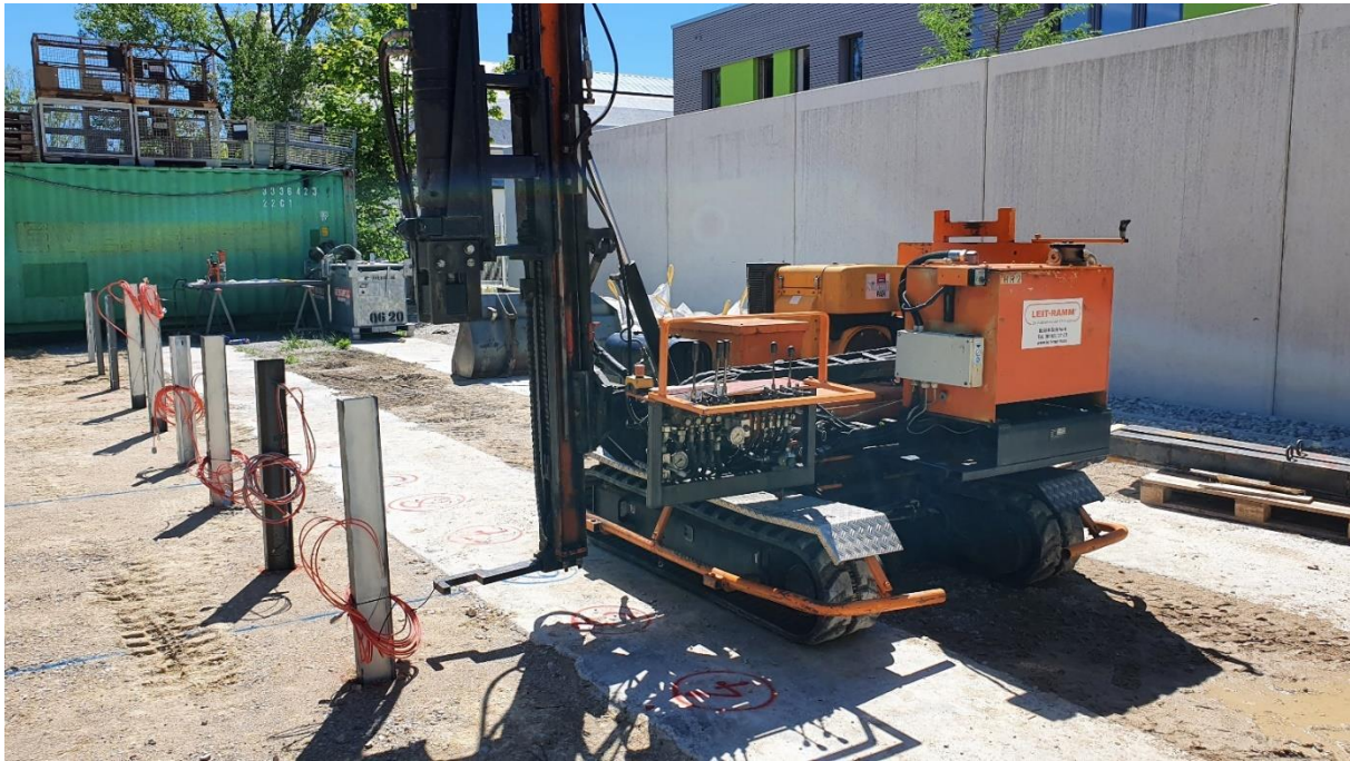
Fig. 3-16: Installation of instrumented posts using a hydraulic guardrail post driver
