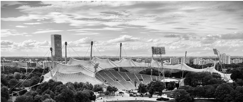
Figure 5.21: Roof of the Olympic Stadium in Munich (on 01.09.2023).
