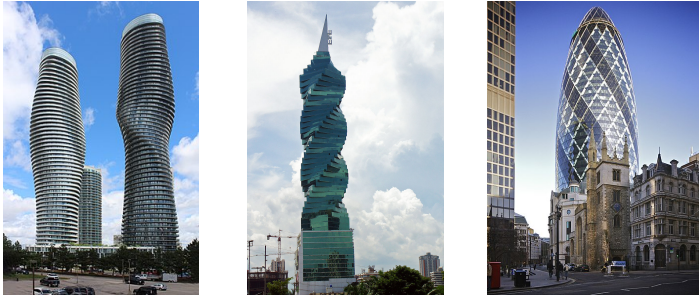
Figure 4.1 : Modern tall buildings with unconventional shapes - Absolute World Towers, Mississauga, Canada have an elliptical cross-section with twist along the height [88] (left); (b) F&F tower, Panama has a twist along the height [89] (middle); and (c) 30 St Mary Axe tower, London has a circular dome at the roof [90] (right).
