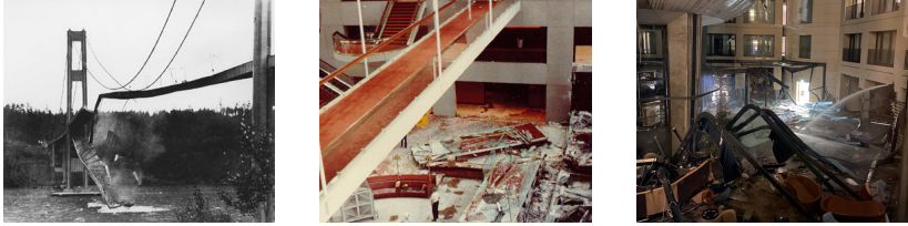
Figure 1.1 : Structural failures have had catastrophic consequences in the past, such as Collapse of the Tacoma Narrows Bridge [2] (left); the tragic collapse of a walkway at the Hyatt Regency in Kansas City in 1981, causing human casualties [3] (middle); and the failure of AquaDom aquarium at hotel Radisson in Berlin 2022 causing around 1500 aquatic life casualties [4] (right).
