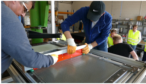
(A) Applying UHPC
