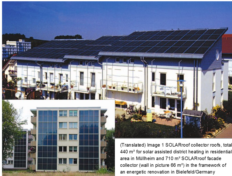
FIGURE 2.2.3. SOLARroof of Wagner & Co, excerpt of technical information from 2007 [161]
