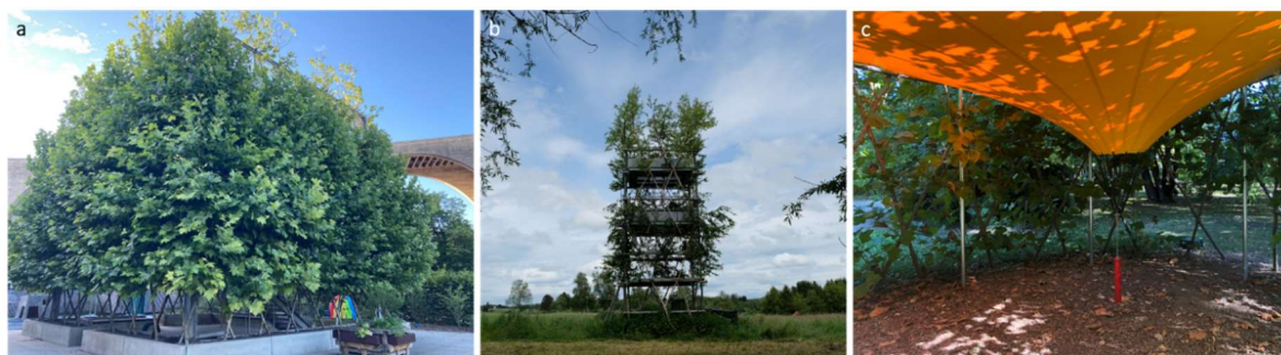
Figure 1.3. Three Baubotanik structures utilising cross-wise inoscultations: (a) the Plane Tree Cube in Nagold (photo: James Barnes), (b) the Baubotanik Tower at Werkpark Neue Kunst am Ried (photo: Ferdinand Ludwig), (c) and the Freiburg Pavilion in Freiburg Botanical Garden (photo: Thomas Speck).
