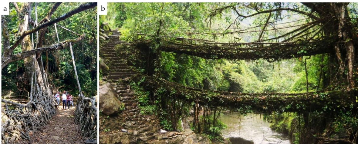
Figure 2.16. (a) Wah Thyllong bridge connecting Nohwet and Riwai villages has a wide and comfortable gangway. (b) A second deck was established on Nongriat Double Decker bridge. According to local residents the upper deck was grown to allow the use of the bridge when the lower deck was flooded (photo: Patrick Rogers).
