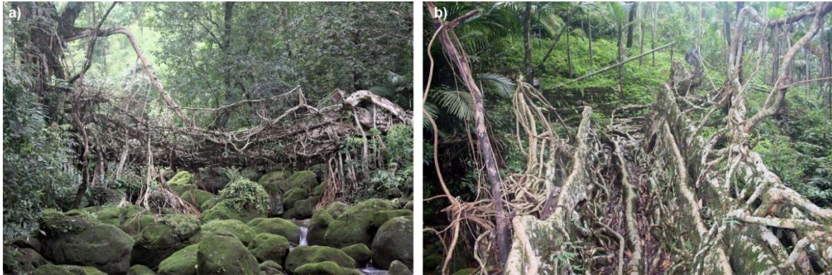
Figure 1.10. Ummonoi bridge with five structurally important roots running the length of the deck and handrails: (a) from downstream, (b) along its length. From Ludwig et al (2019) [74] .
