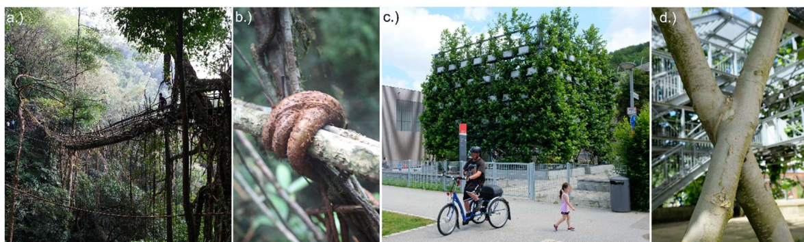
Figure 3.1. Living architecture exhibits points of interest on a range of scales: (a) a 53m long living root bridge (photo: W. Middleton), (b) details in bridges are at the cm scale (W. Middleton), (c) the Nagold Plane Tree Cube, a contemporary Baubotanik example (F. Ludwig), (d) an inosculation in the Plane Tree Cube (F. Ludwig).
