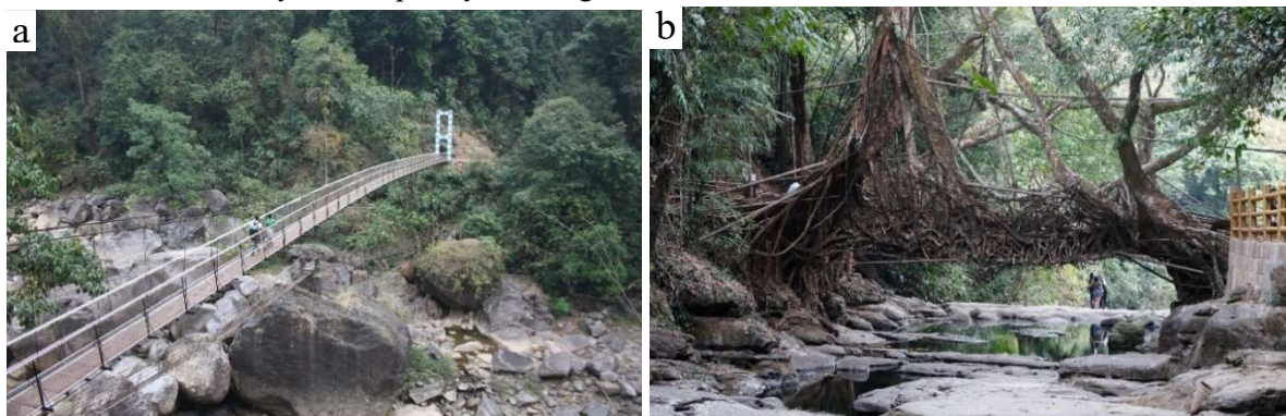
Figure 2.5. Two contrasting aesthetics: (a) the steel bridge towards Nongriat village can be described as modern, efficient and professional; (b) the traditional Wah Thyllong bridge can be seen as an example of the Ecological Beauty of LRBs. The bank reinforcement and railing made of imported Cherra stone and painted reinforced concrete (imitating bamboo) illustrate a break with this tradition.
