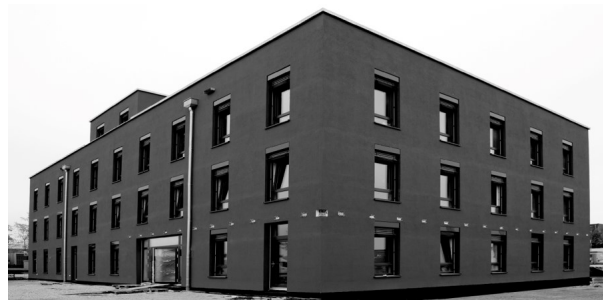
Figure 3.19: Ferdinand Tausendpfund GmbH & Co. KG office building, in Regensburg, Germany built in 2017. It has three storeys and is 27m long, 14.7m wide, and 9.8m tall. The gross volume is approx. 3950 m 3 , with a gross area of 1290.5 m 2 and a window-to-wall ratio of 25%
