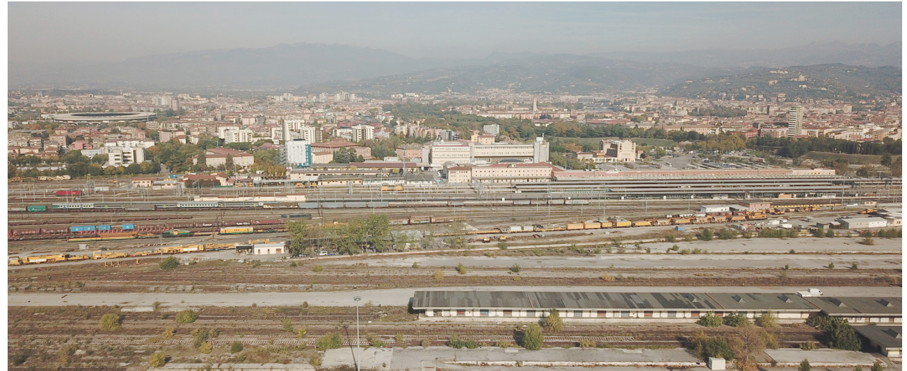
Drone photo of the former freight yard, Porta Nuova
