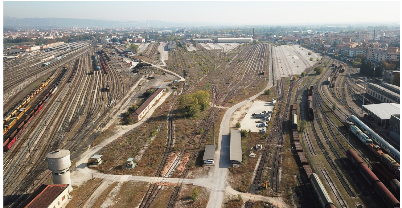
Drone photo of Porta Nuova; East view
