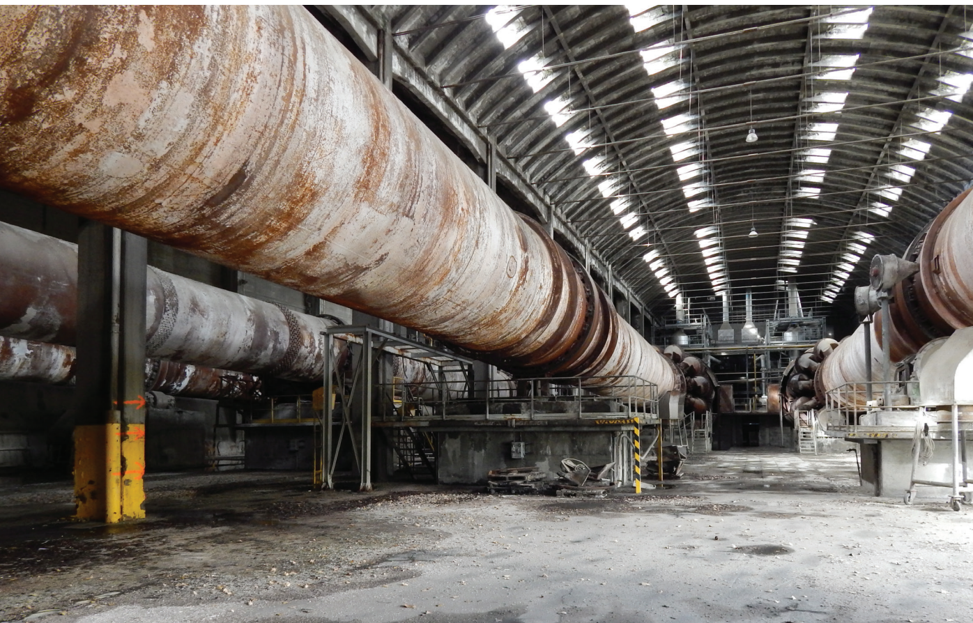
The rotating ovens are one of the most characteristic remnants of the former cement plant
