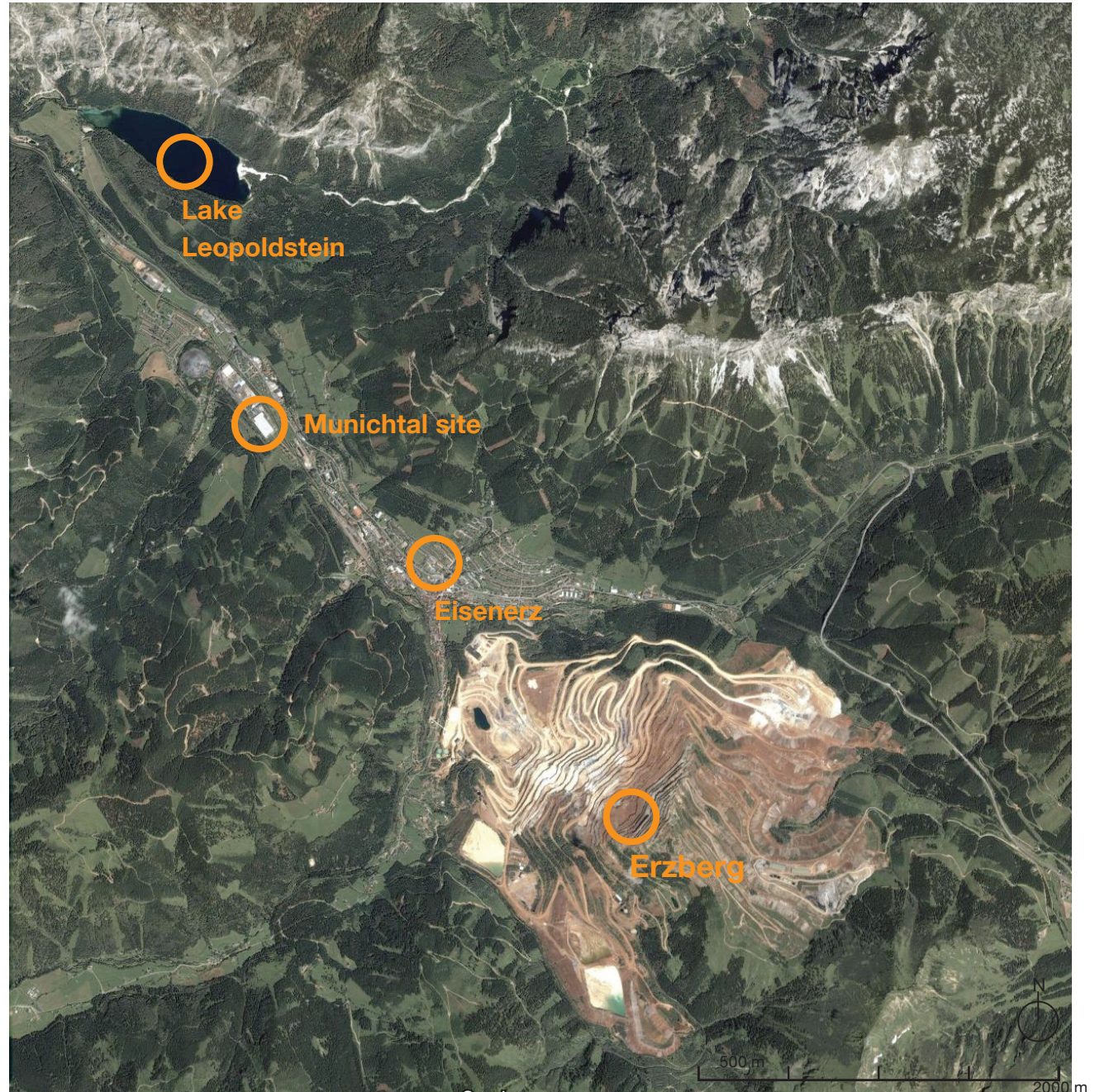
The site is located between Lake Leopoldstein and the city of Eisenerz. The Erzberg with its open-cast iron ore mine, which is still in use, borders the city of Eisenerz in the north. Therefore the city is an important link between the iron ore mine and the brownfield site.
