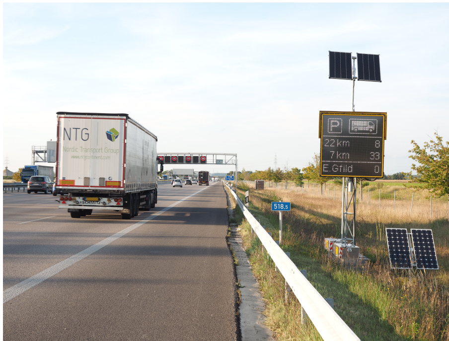
Figure 2.5: Research project truck parking availability dissemination via VMSs on the A9 - source: Lukas Kremtz
