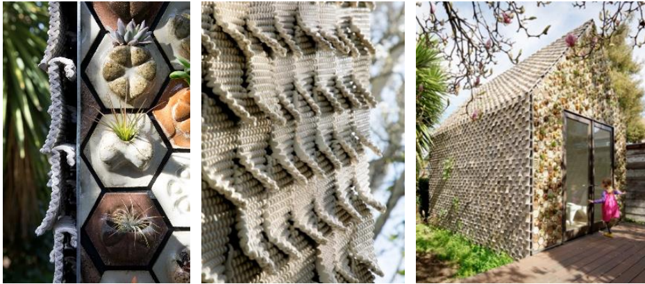
Figure 8: digitally fabricated clay facades with greenery integration of “Cabin of curiosity”, Emerging Objects Studio
