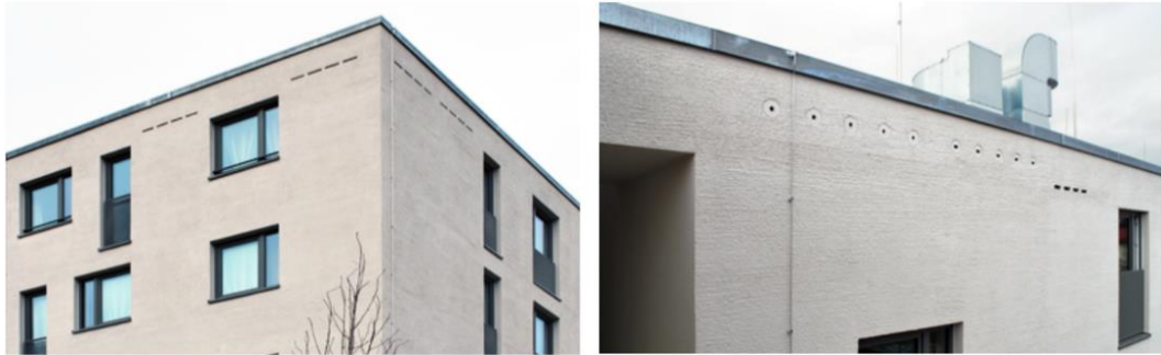
Figure 5: Integration of nests into buildings' facades, Weisser & Hauck
