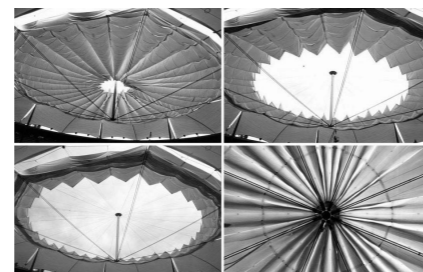
Fig. 5: Sequential view of membrane roof
