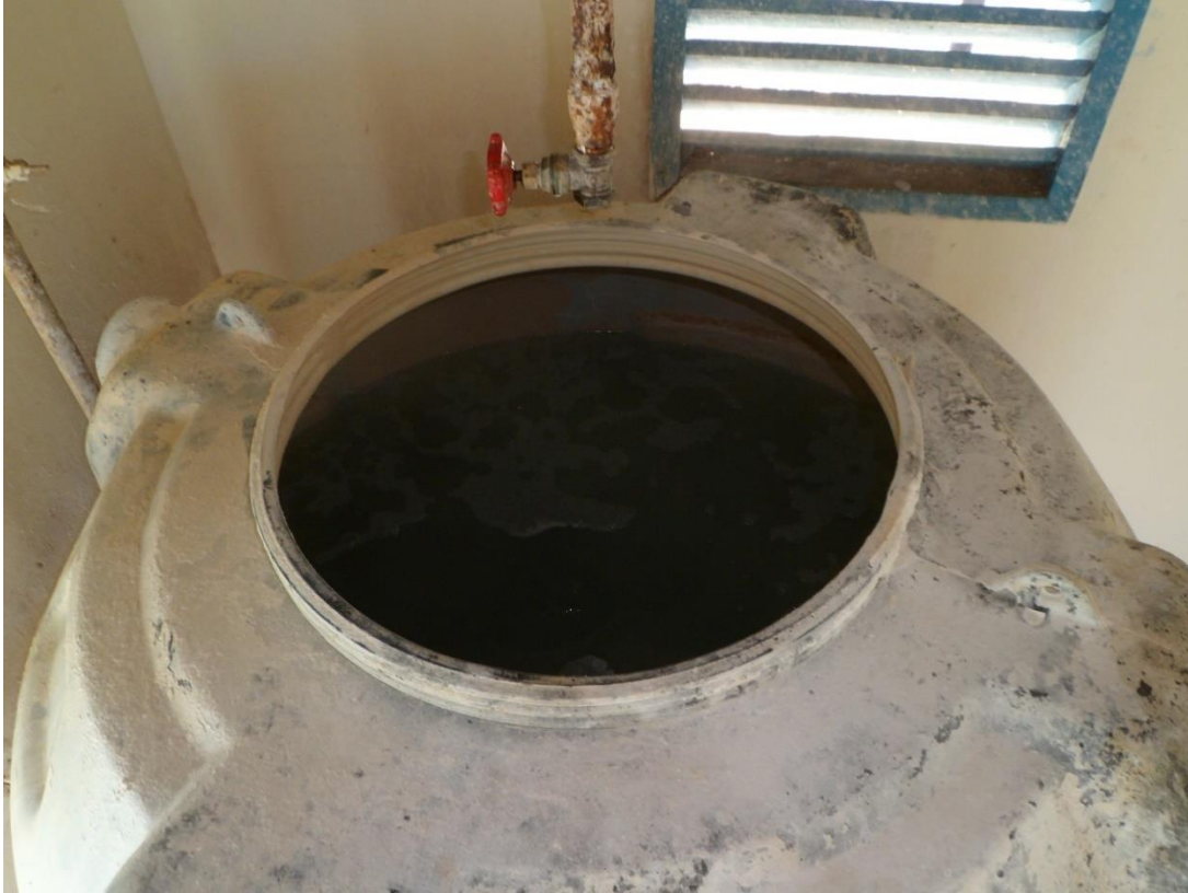
lxxxii) Top view of the chlorine tank in which the disinfectant solution is prepared and stored before it is dosed to the water stream. The chlorine species applied is high test hypochlorite (HTH).
