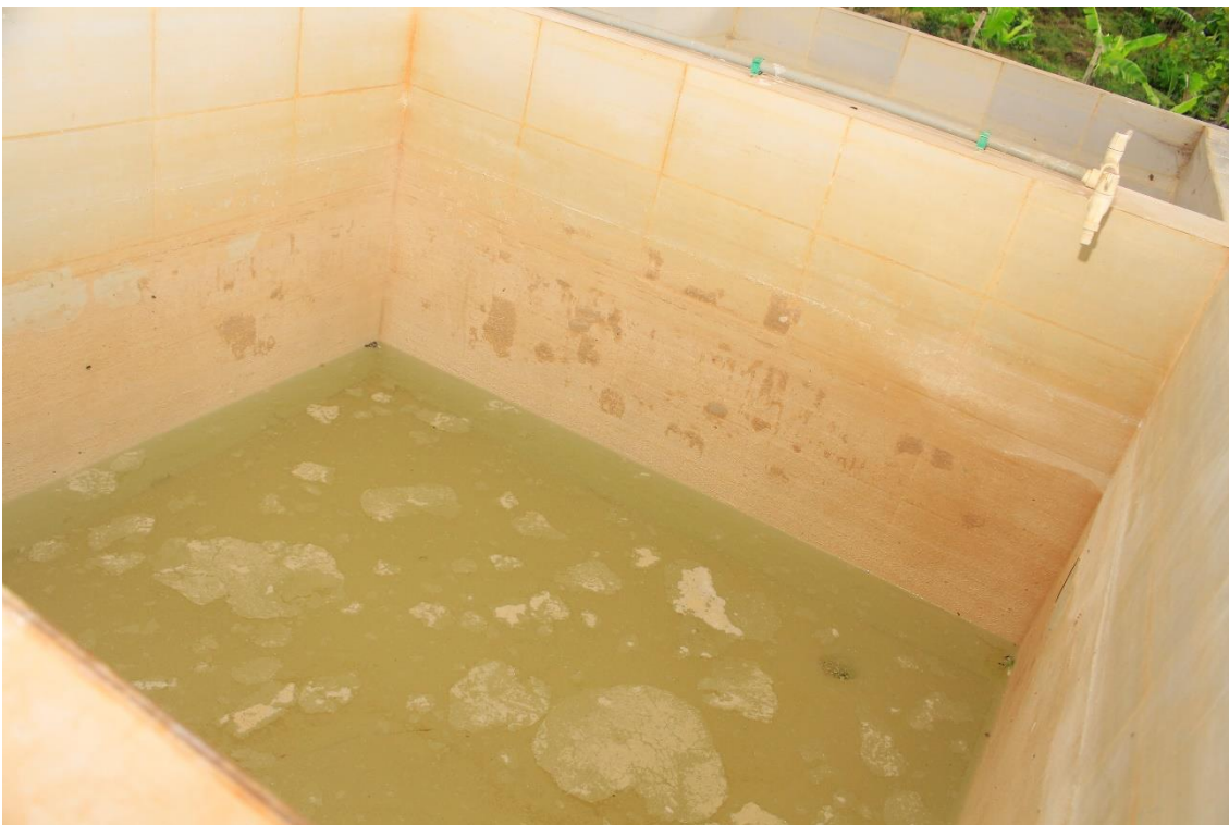
xxxi) Chlorine solution in the chlorine tank. The chlorine species applied is high test hypochlorite (HTH). Photo by Elias Okemer.
