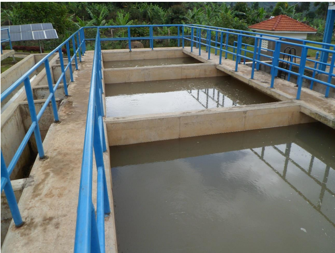
xxvii) After sedimentation, the water is filtered in a rapid sand filtration system.
