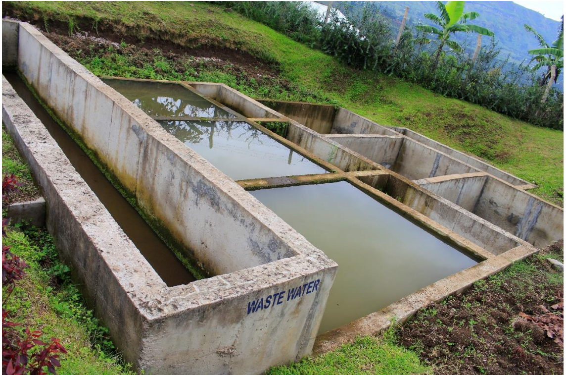
xi) Drying beds for the treatment of wastewater generated during drinking water production, mainly from backwashing and cleaning of clarifiers. Photo by Elias Okemer.
