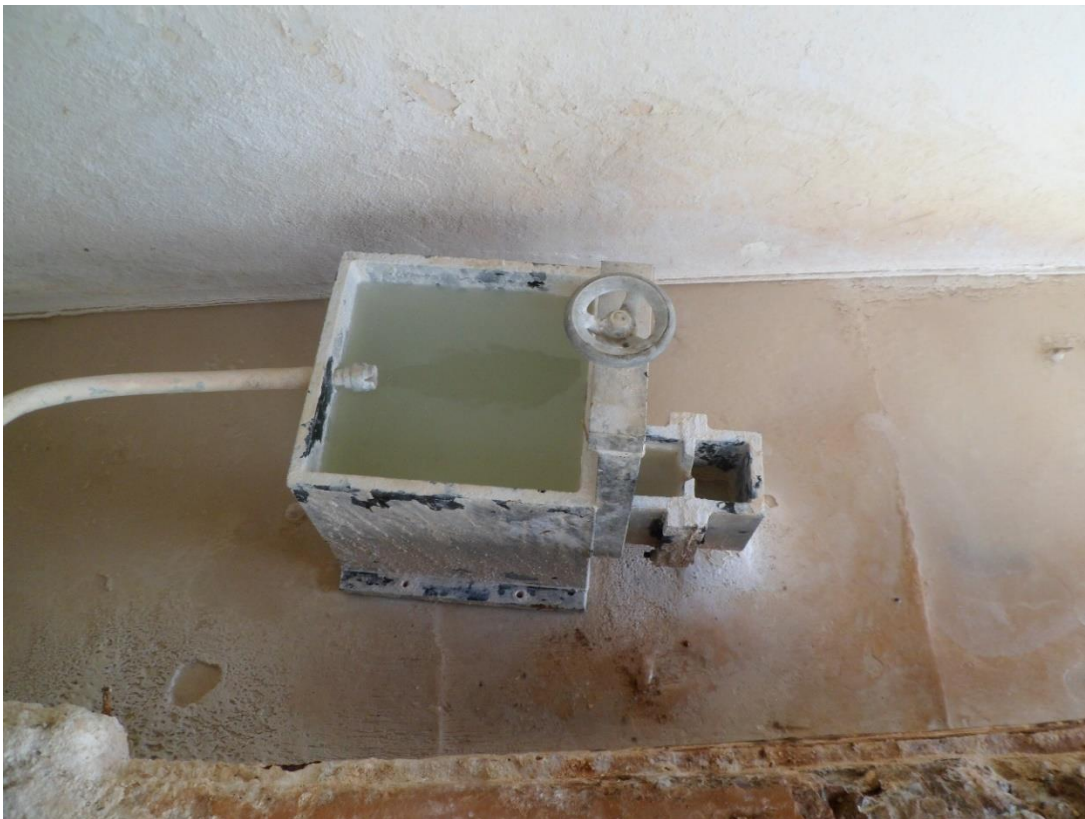
lxxxiii) The dosing device applies the disinfectant solution through the floor of the chlorine room to the water stream that enters the final water tank after filtration.
