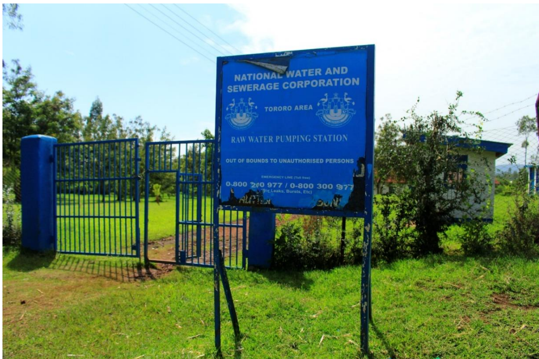
ixi) Signpost of the raw water pumping station of Malaba-Tororo Water Supply (referred to as "Malaba-Tororo") in Tororo district, eastern Uganda. Exact location: 0°37'31.7"N 34°12'24.8"E. Photo by Elias Okemer.
