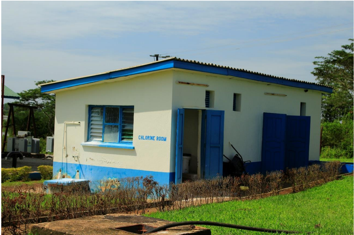
lxxvi) Operations building for the chlorine dosing and backwashing systems. Photo by Elias Okemer.
