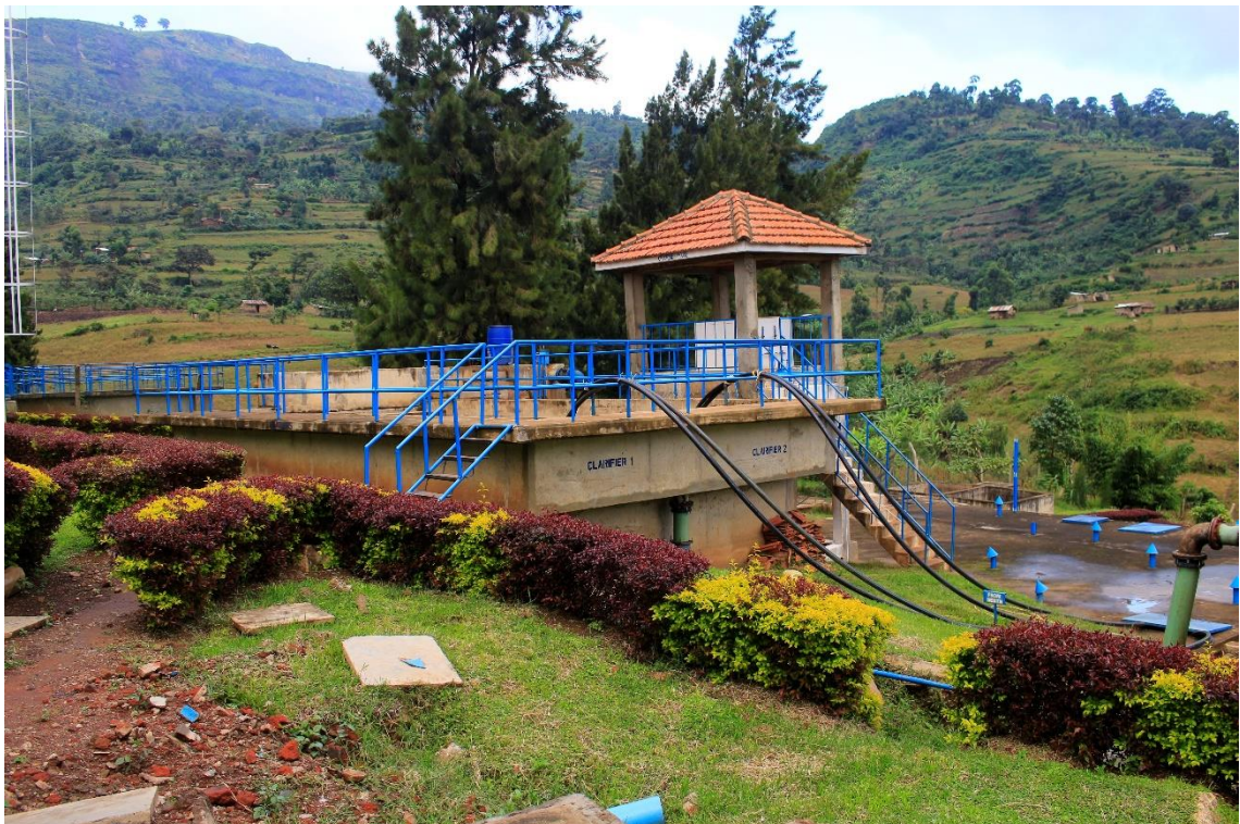
xlv) Overview of the DWTP of Sono. Sedimentation stage (clarifiers 1 and 2) in the centre of the picture, behind it the chlorine tank for disinfectant dosing located under the roof. On the right is the clear water well for the final water. Photo by Elias Okemer.
