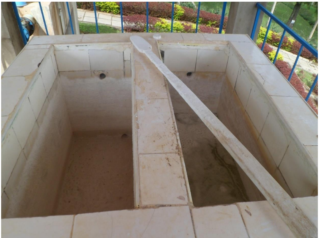
liii) Chlorine solution in the chlorine tank. The chlorine species applied is high test hypochlorite (HTH). The disinfectant solution is dosed directly to the clear water tank.
