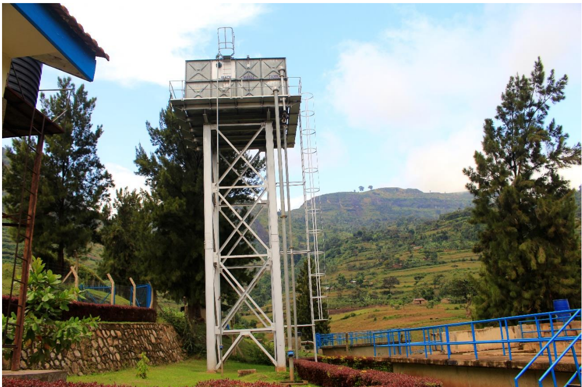
lvii) Elevated backwash water tank. Like at Lirima, final water is withdrawn from the clear water well and pumped by backwash pumps to the elevated tank. During backwashing, water flows by gravity from the backwash water tank to the sand filters. Since the filters were not in operation at the time of the site visit, the backwashing system was not used as well. Photo by Elias Okemer.
