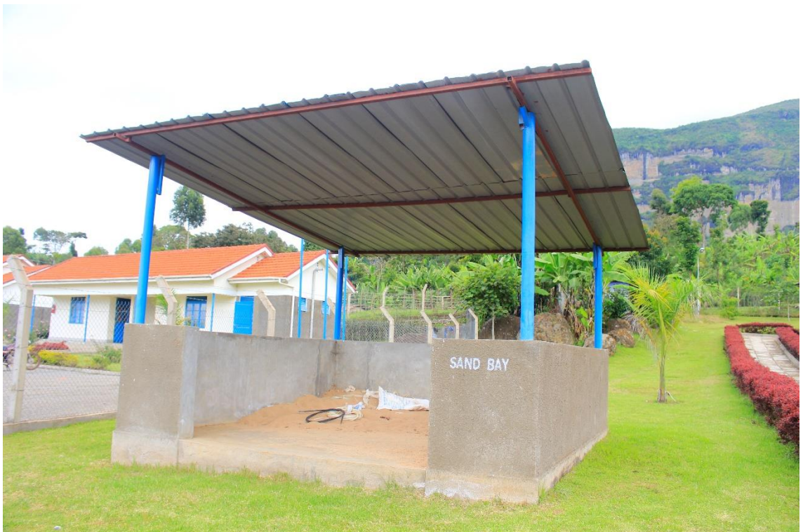
xii) Sand bay for storing of filter sand. Photo by Elias Okemer.
