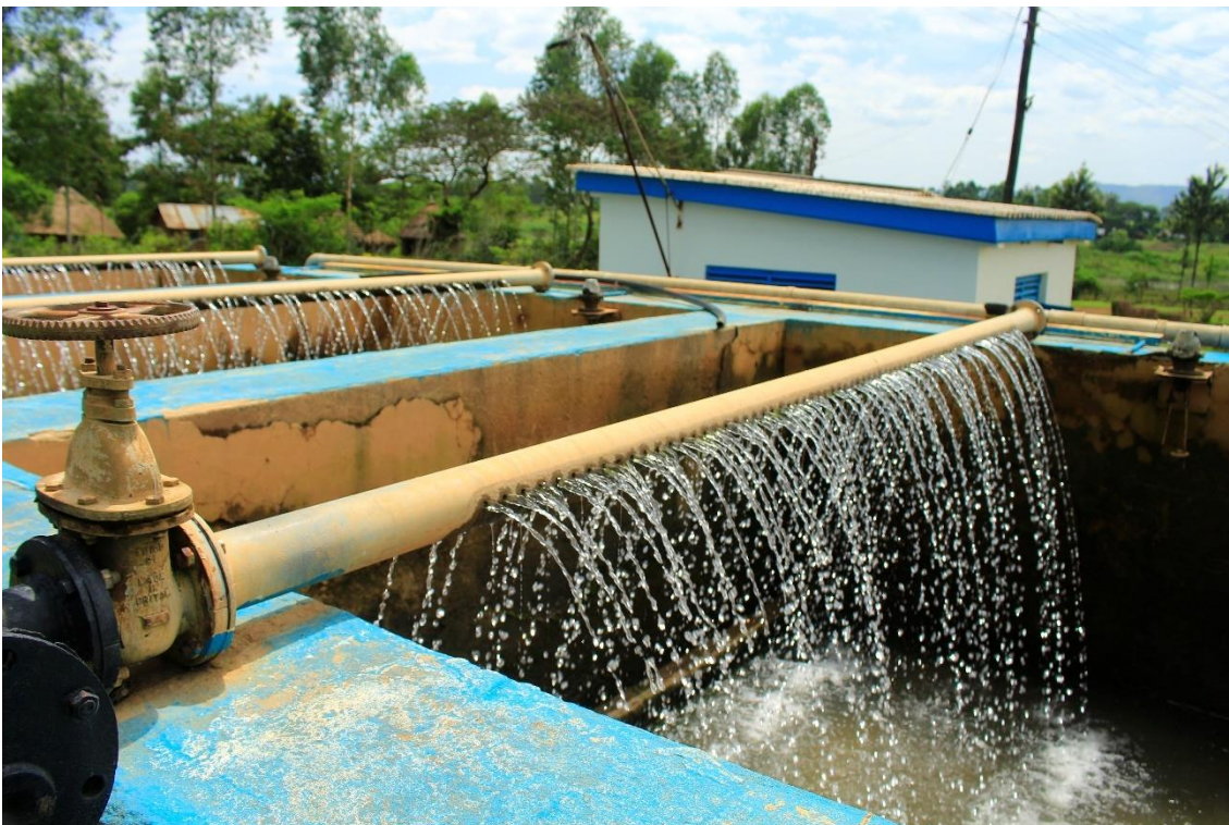
lxxv) Rapid sand filtration at the old line of the DWTP. Photo by Elias Okemer.
