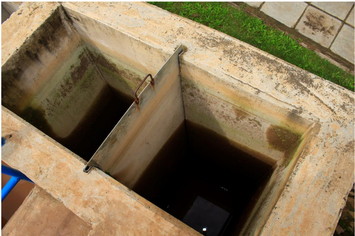
xlix) After dosing of the coagulant, the water flows into these flocculation chambers. The treatment stage is designed considerably smaller compared to the hydraulic flocculation system at Lirima. According to the plant overseers, it does not provide sufficient time for the coagulant chemical to mix and react with the water. Therefore, flocculation cannot take place properly. After the flocculation chambers, the water enters the clarifiers. Photo by Elias Okemer.
