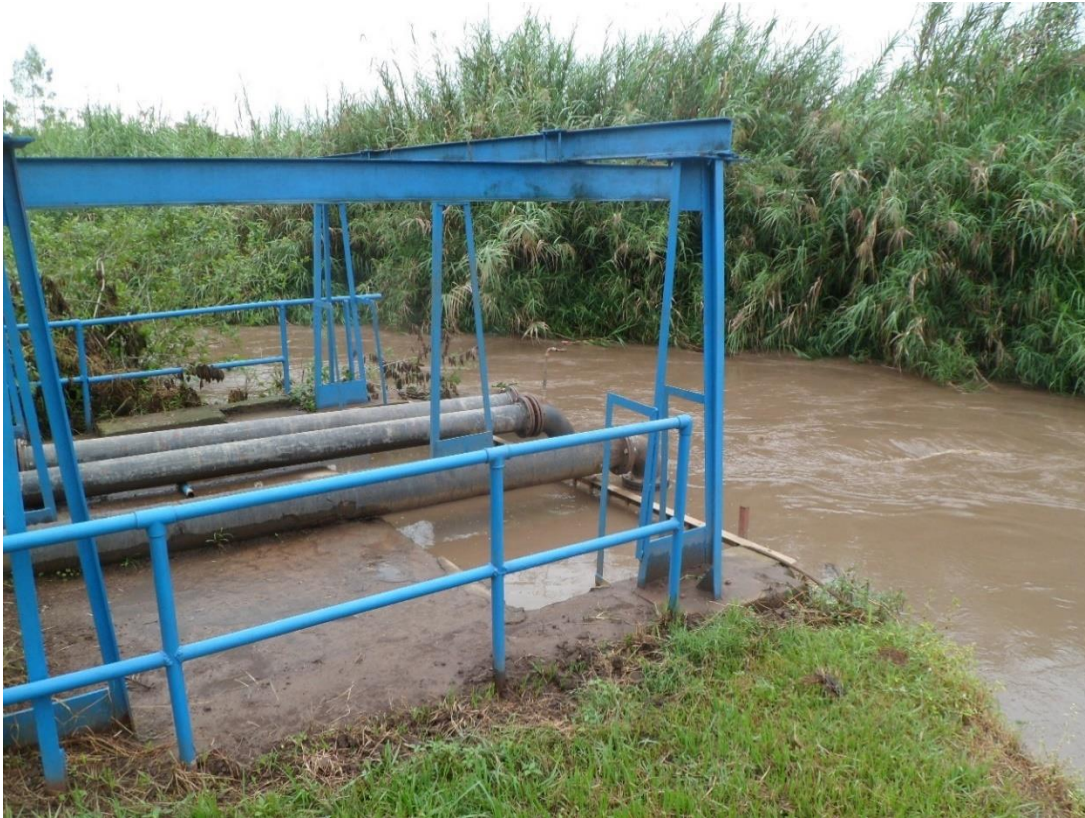
lxii) Raw water intake of Malaba-Tororo, located in the lower reaches of river Malaba. In the area, the stream constitutes the national border of Uganda and Kenya. The stream water appears muddy, silty, and turbid.
