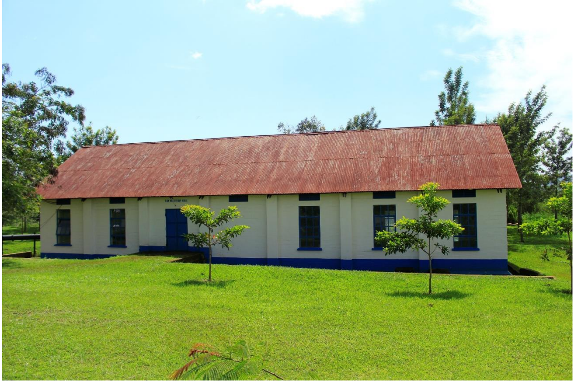
lxiv) Pump house for raw water pumps, coagulant dosing, and coagulant storage at Malaba-Tororo. Photo by Elias Okemer.
