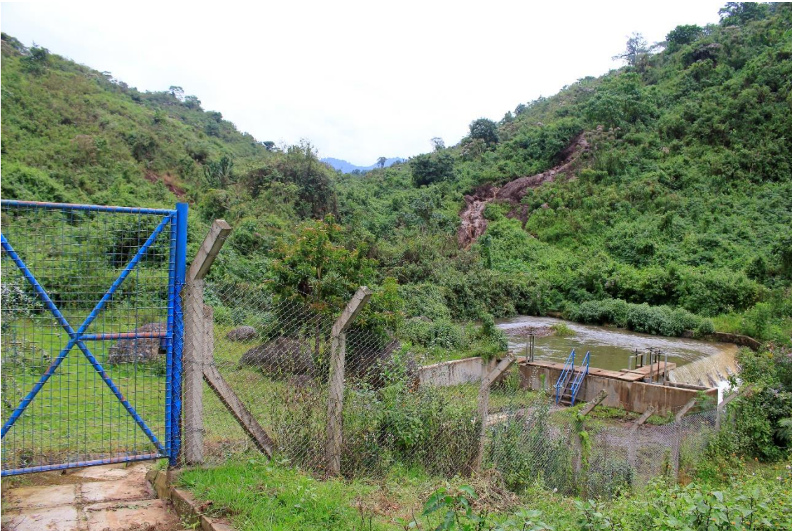
xix) Raw water intake of Lirima Gravity Flow Scheme, located in the course of river Lirima. The area is fenced off to protect the surrounding natural vegetation from human activities. This reduces the inflow of sediments into the intake structure. Exact location: 0°54'08.6"N 34°25'04.5"E. Photo by Elias Okemer.
