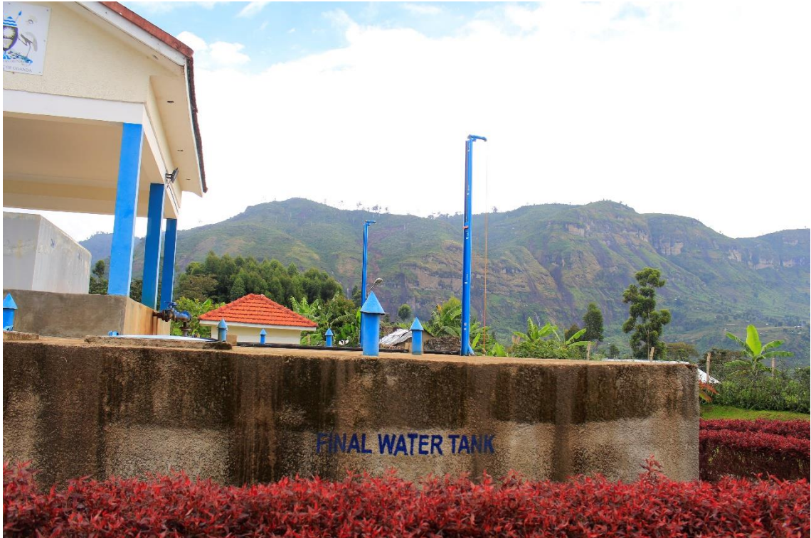
xxxii) Final water tank with water level meters. Photo by Elias Okemer.
