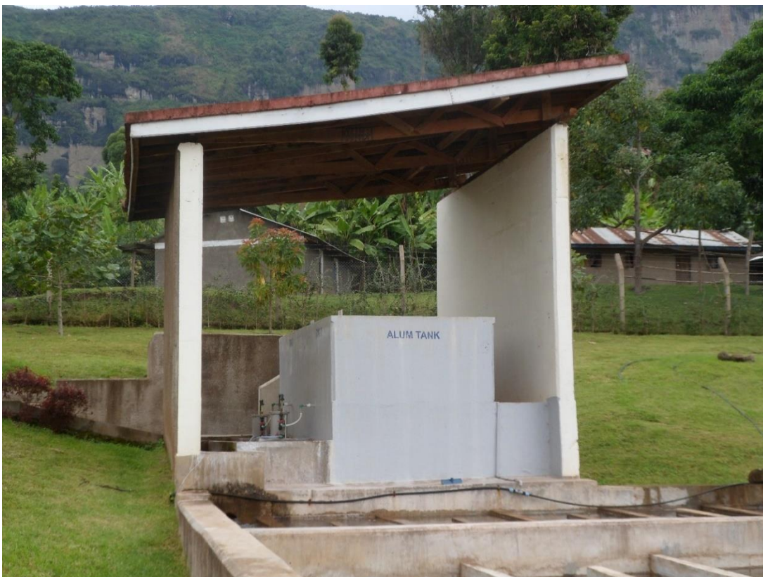
xxiii) In the alum tank, a coagulant solution is prepared by mixing aluminium sulphate ("alum") with water. The coagulant solution is then dosed to the inflowing, turbulent raw water stream.
