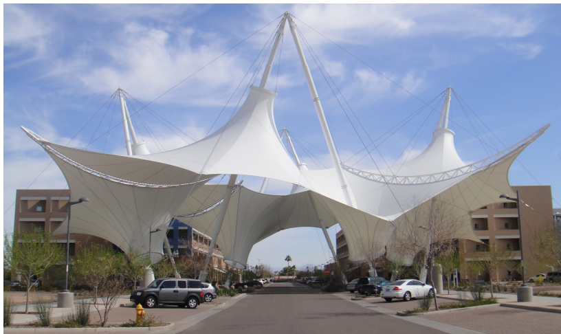
Figure 4.9: The skysong membrane structure in Arizona, USA, adapted in size. ©Cygnusloop99.
