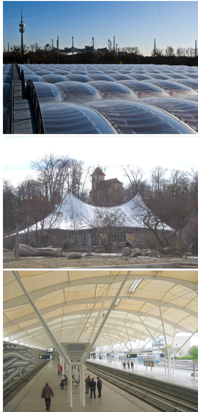
Figure 2.1: Membrane roofs in Munich. Top: Photovoltaic ETFE cushions at the municipal waste management department (©MdCALmeida Villafuerte). Middle: Hellabrunn Zoo: ETFE roof over jungle tent. Bottom: Fröttmaning subway station (©Florian Schütz).
