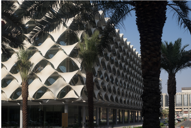
Figure 4.12: King Fahad library with a modular membrane facade. ©Mrcosch.
