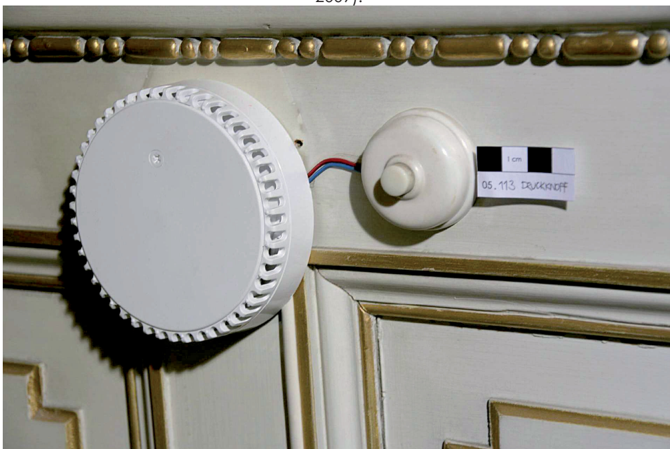
5.113/12 Moderne Installationselemente links neben Tür zu 05.114 (Edlmann 2009).
