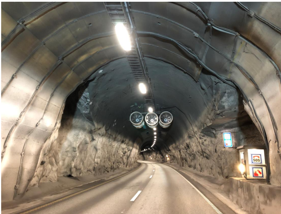
Figure 10-65 : PE-isolation mounted on the rock surface. Fløyttunnel, Norway
