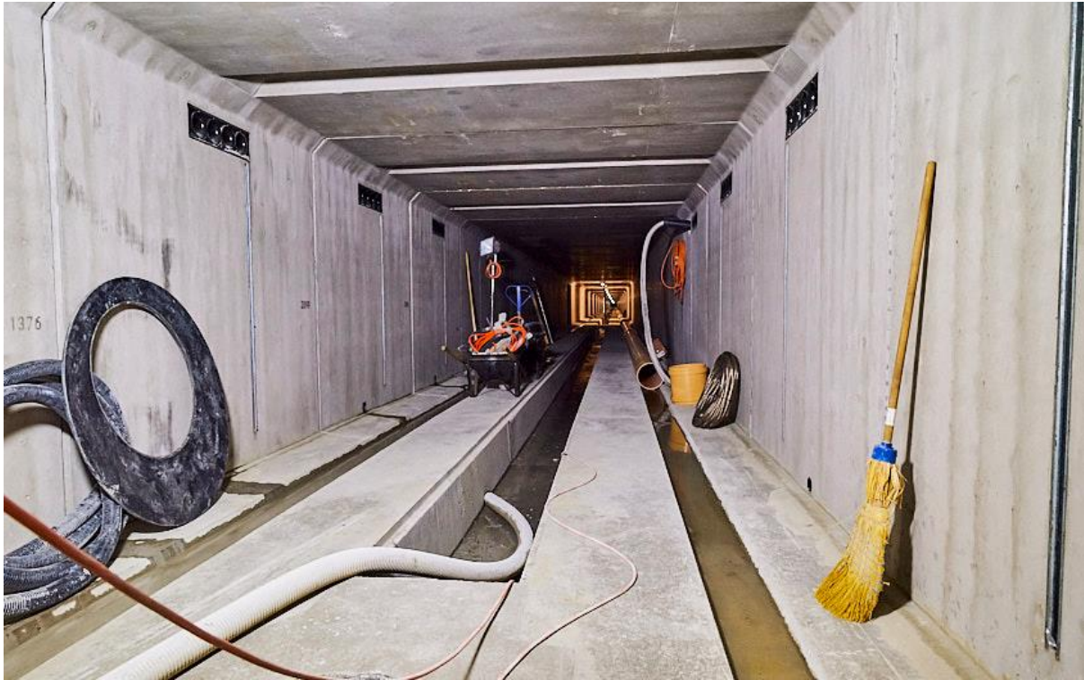
Figure 10-72 : Service gallery under carriageway (source ARGE Marti Belchen)
