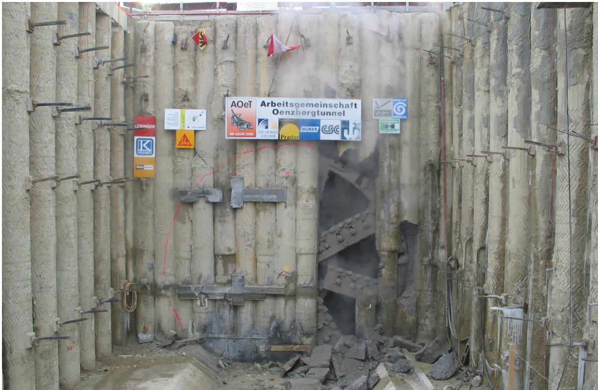
Figure 10-50 : Anchored bored pile wall (source ILF)
