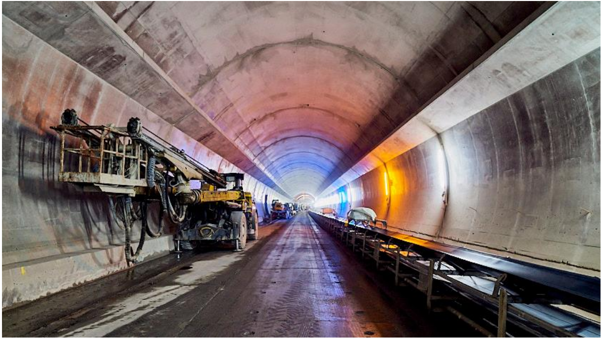
Figure 10-70 : Inner lining with ceiling supports (source ARGE Marti Belchen)
