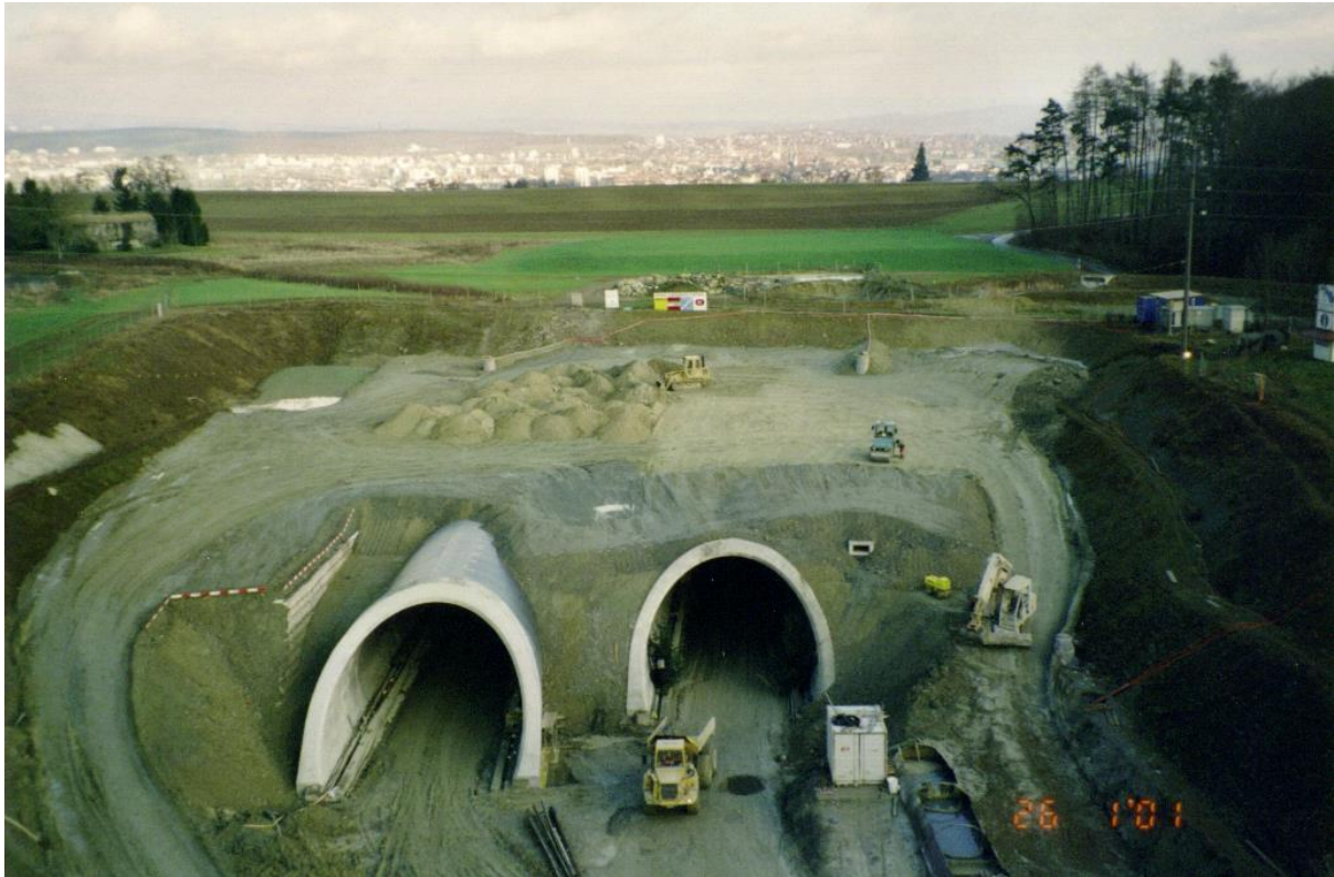
Figure 9-6 : Cut and cover construction in an open excavation (source ARGE Girsbergtunnel)
