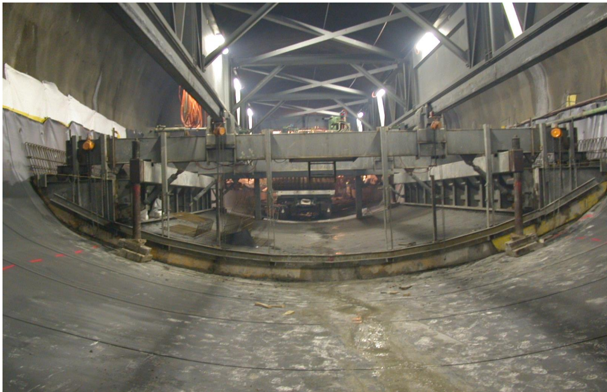
Figure 10-73 : Invert arch lining (source Electrowatt Engineering Services)
