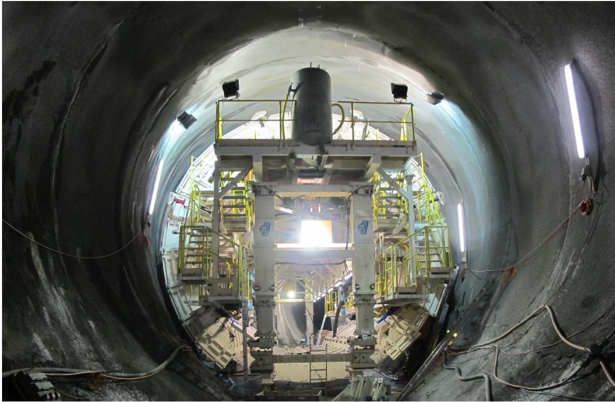
Figure 10-74 : Full round lining formwork in hydro tunnel (source ILF)
