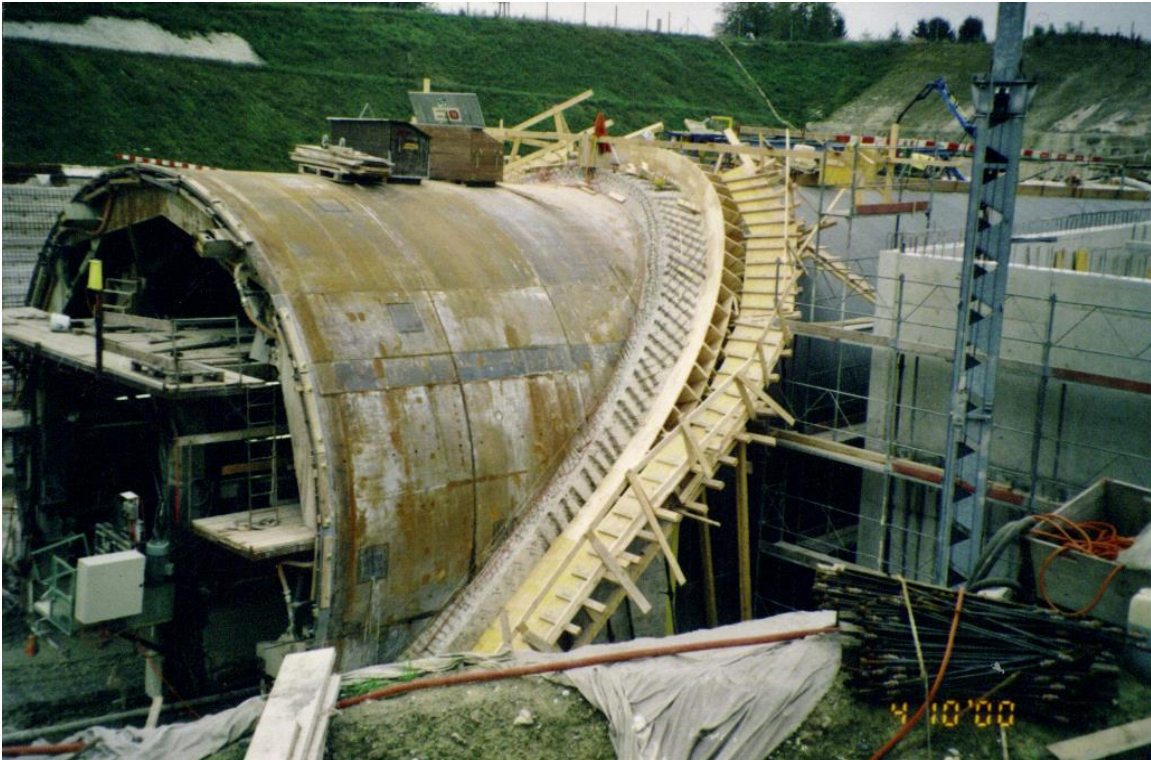
Figure 10-82 : Portal formwork (source ARGE Girsbergtunnel)
