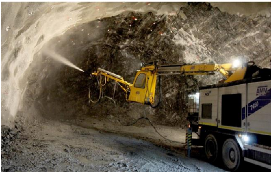
Figure 10-22 : Shotcrete work at face in a Norwegian tunnel.
