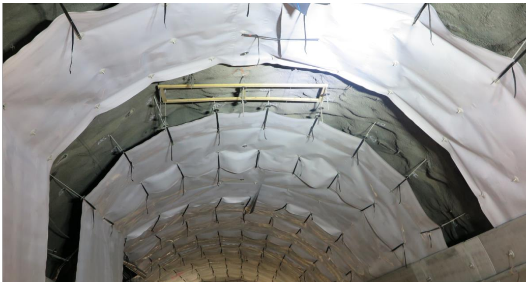
Figure 10-57 : Membrane before shotcrete is applied, Lyshorn tunnel, Norway
