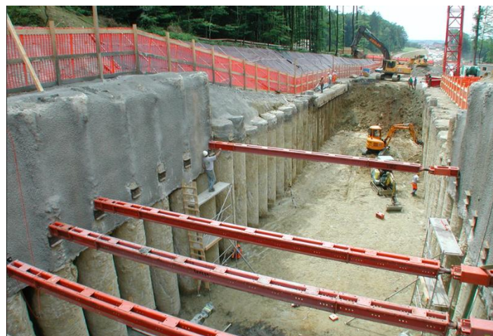
Figure 10-49 : Bored pile wall with bracing (source ILF)
