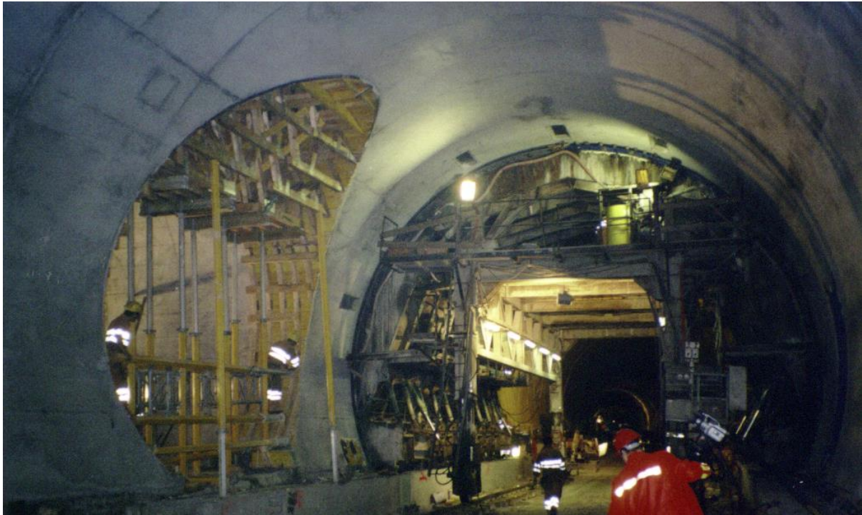
Figure 10-76 : Inner lining formwork (source ARGE Girsbergtunnel)
