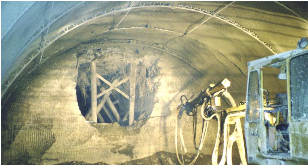
Figure 10-25 : Lattice girders and shotcrete support (source ARGE Girsbergtunnel)
