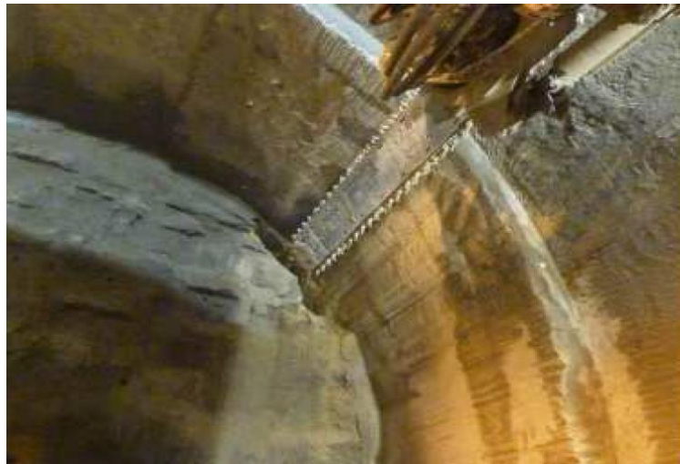
Figure 10-3 : PERFOREX method (source : Insa Lyon, ENTPE, France)
