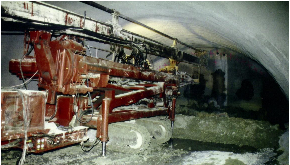
Figure 10-6 : Sub-horizontal jet grouting (source ARGE Girsbergertunnel)
