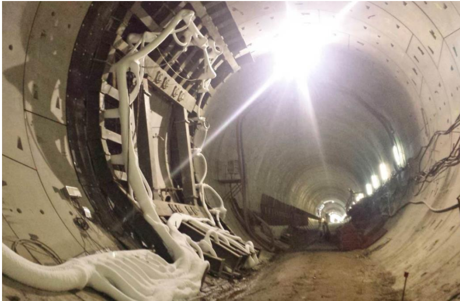
Figure 10-53 : Ground freezing in mechanised tunnelling in Slovacki Tunnel (Poland), courtesy Rodio
