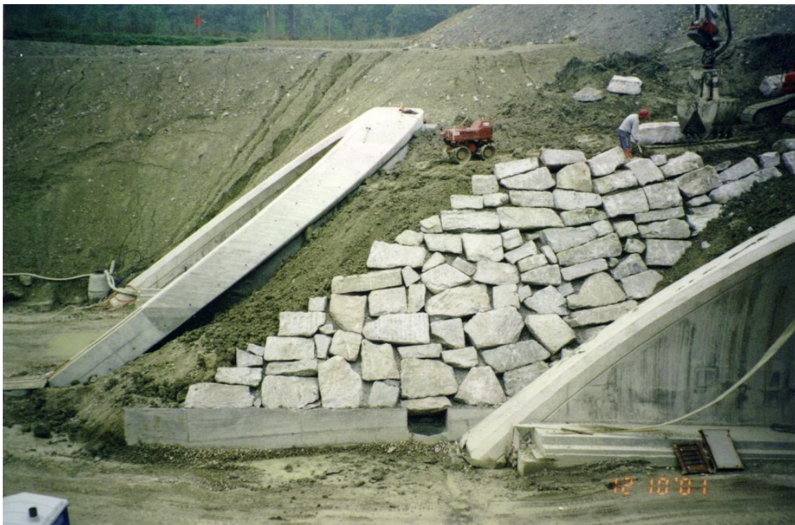
Figure 10-83 : Portal fill and landscaping (source ARGE Girsbergtunnel)
