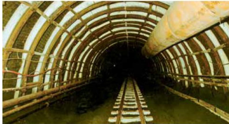
Roof Support Backfilling
