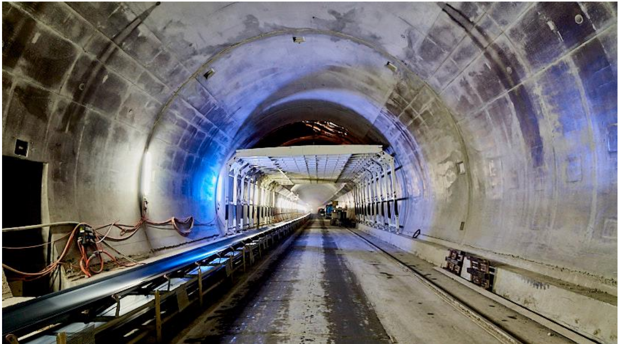
Figure 10-71 : Ventilation ceiling formwork (source ARGE Marti Belchen)
