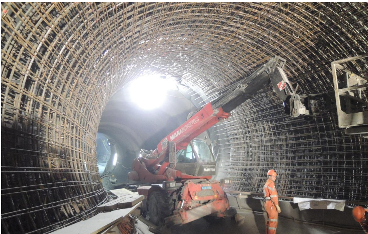
Figure 10-75 : Heavily reinforced tunnel lining (source ILF)
