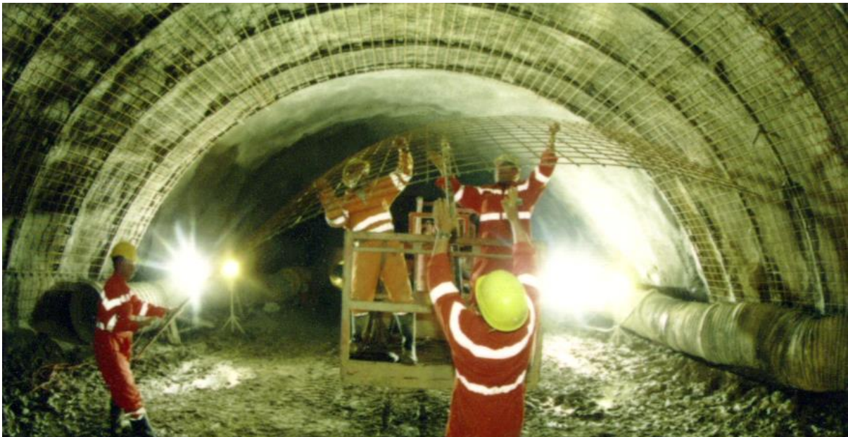
Figure 10-24 : Mesh reinforcement (source ARGE Girsbergtunnel)
