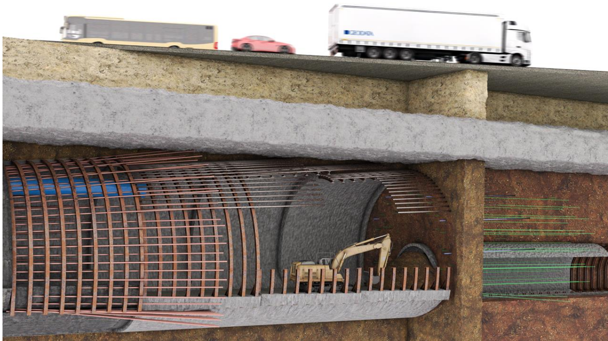
Figure 10-8 : Conventional excavation with forepoling (courtesy Geodata)
