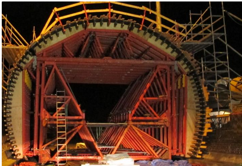
Figure 10-27 : Wagon for casted inner lining, Knappe Tunnel, Norway
