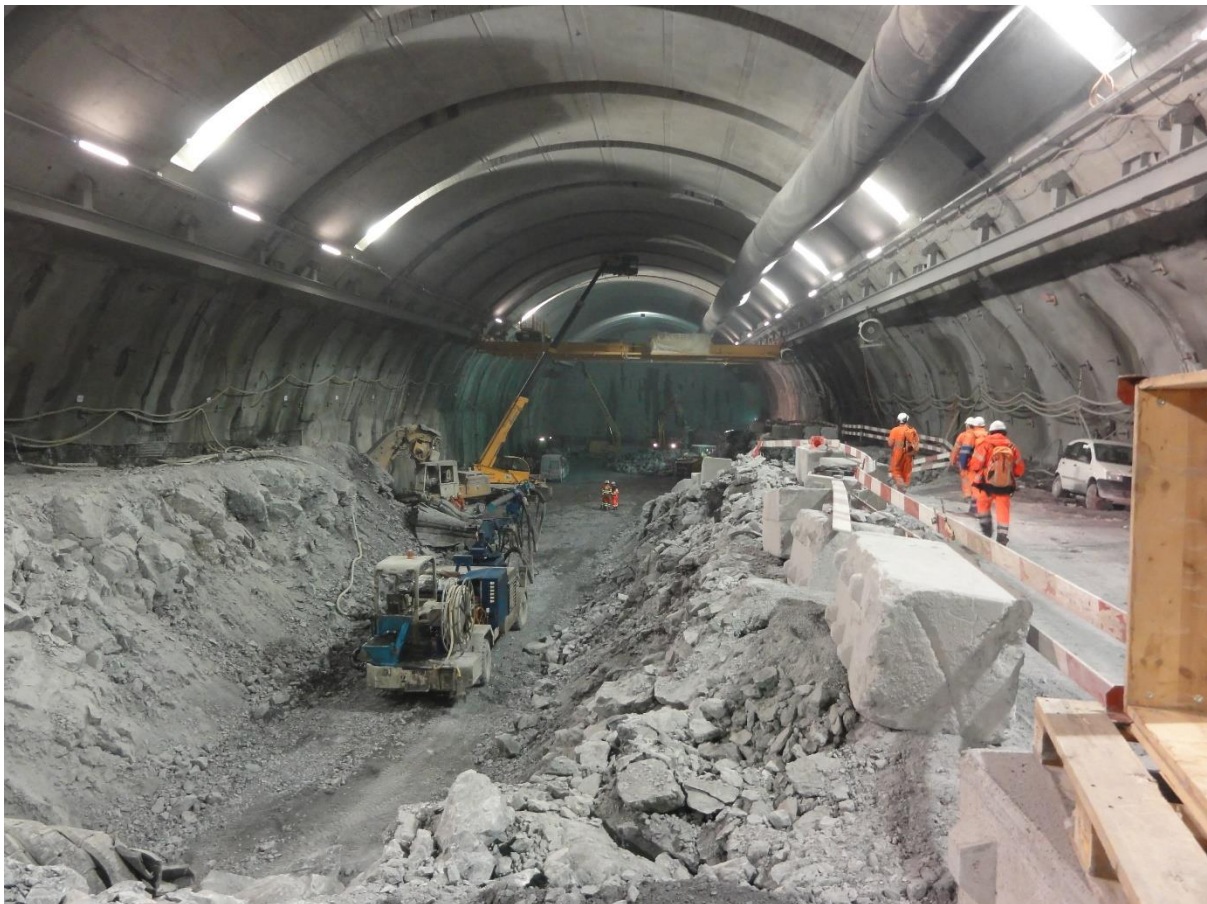
Figure 9-2 : Staged cavern excavation by drill and blast (source ILF)
