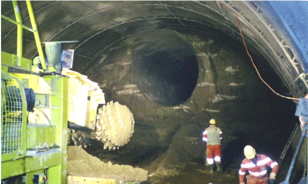
Figure 9-1 : Excavation with road header and ventilation pilot tunnel (source ARGE Girsbergtunnel)
