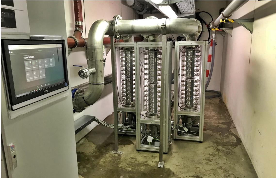
**Figure 10.1:** Photograph of the full-scale US reactor system depicting individual reactors, pipes, and the control cabinet at the Starnberg wastewater treatment plant.
