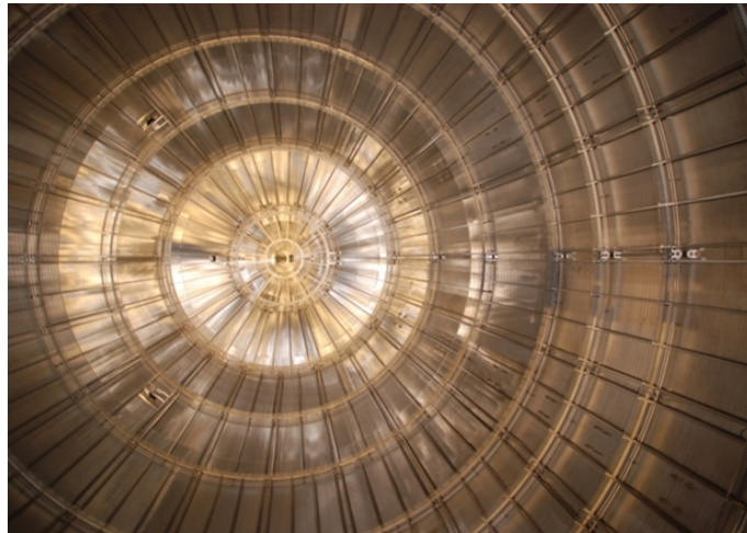
Figure 4.11: The inner surface of the MS is covered by an IE system. Being on more negative potential than the vessel hull, electrons created at the surface are guided back to the walls.
