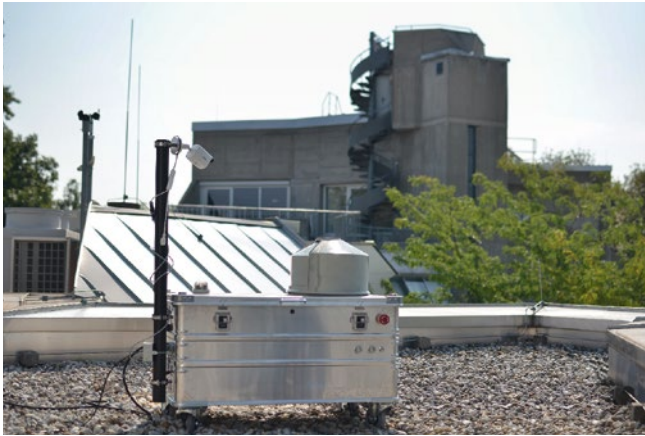
1 | GHG measurement system on top of the roof of MPE Garching (© Andreas Forstmaier)
