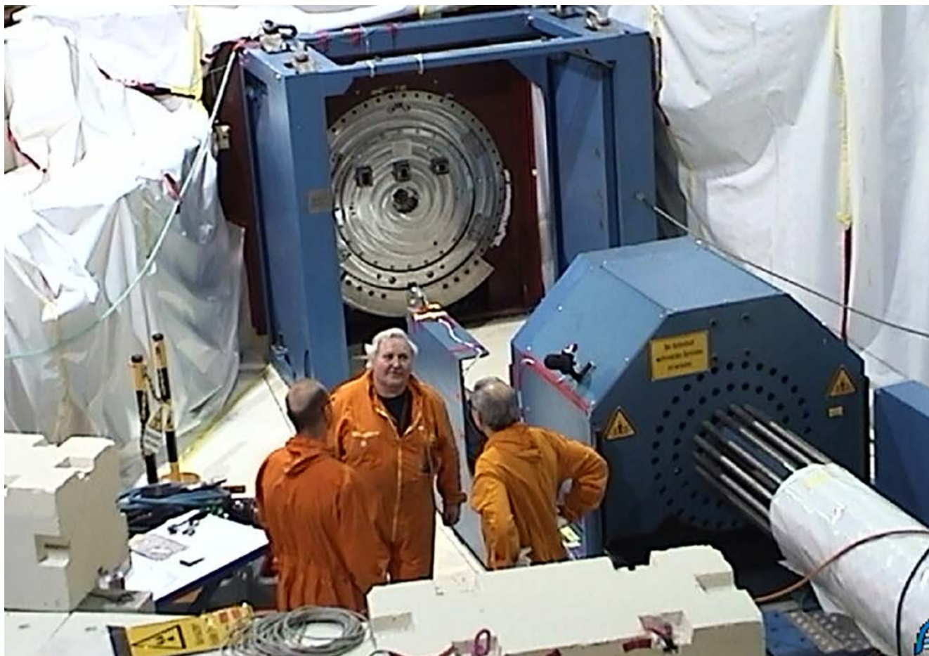
Figure 4: The new plug JMA05 after its successful assembly in the beam tube SR5. This represented the end of the hot phase of the replacement of plug JMA05.
