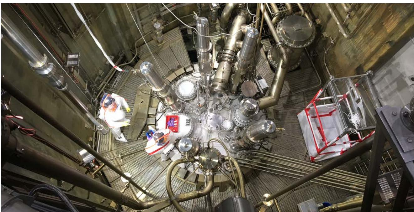
Figure 3: The thimbles in the reactor pool were exchanged for newly manufactured parts.
