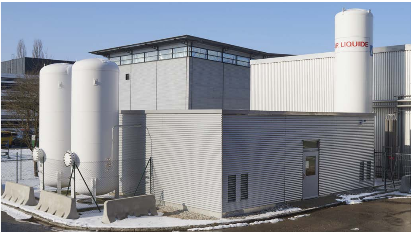
Figure 1: Newly built housing to the south of the MLL for the He-compressors of the UCN-source, with two helium gas tanks (on the left) and a liquid nitrogen tank (on the right).
