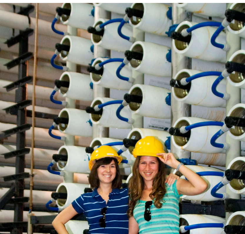
Figure 1: Ashkelon Seawater Desalination Plant (Israel) using Reverse Osmosis (RO) Technique. Produces 330,000 m 3 potable water per day for 0.57 $/m 3 . The two young ladies are former students of the Zuckerberg Institute for Water Research.
