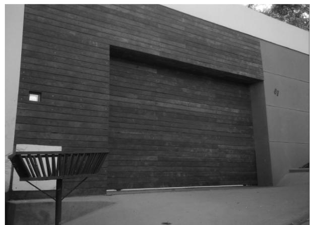
Figure 4: Plastic timber facade coating – image courtesy of Ecoblock company
