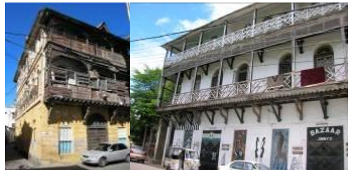
Fig 7: Views of Houses with a balcony that spans two floors in old town Mombasa.
