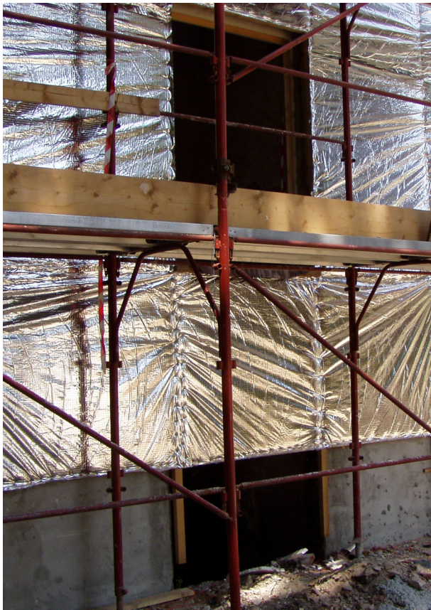
Figure 9: Thin insulation used in the retrofitting.
