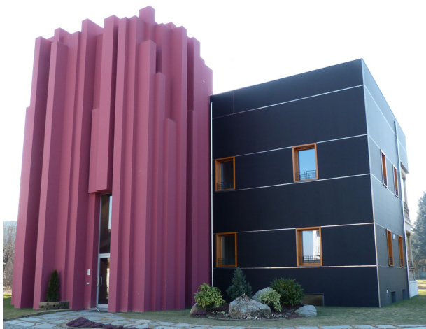
Figure 5: North view of the building after the restoration.
