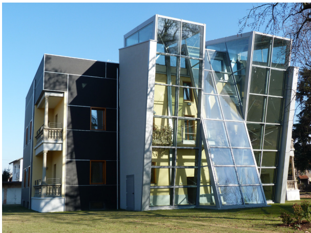
Figure 3: South view of the building after the restoration.
