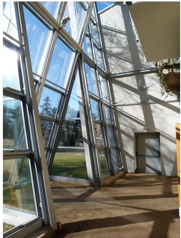
Figure 8: Interior view of the greenhouse.
