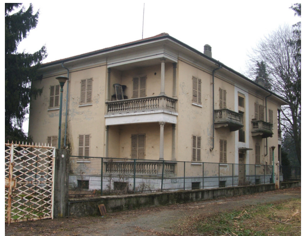
Figure 2: The building of the ex CRE at Chivasso just before retrofit.
